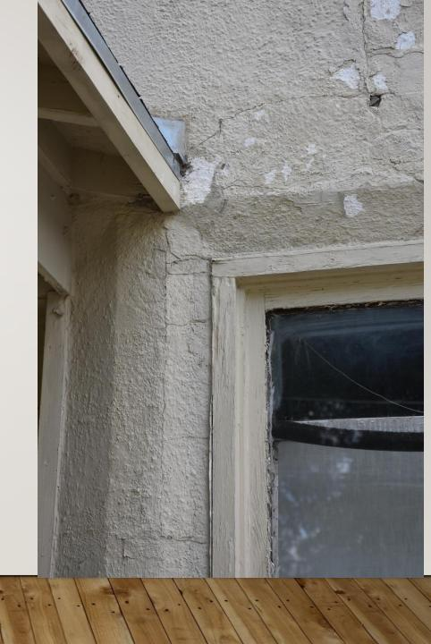
Ponding water and likely wood framing deterioration and decay behind the stucco (red circles)
