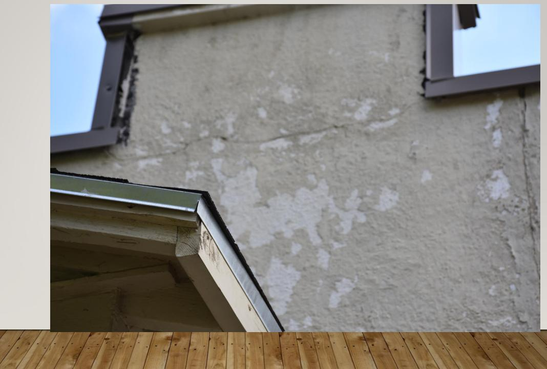
Evidence of water infiltration throughout the cladding indicating a high likelihood of wood deterioration
