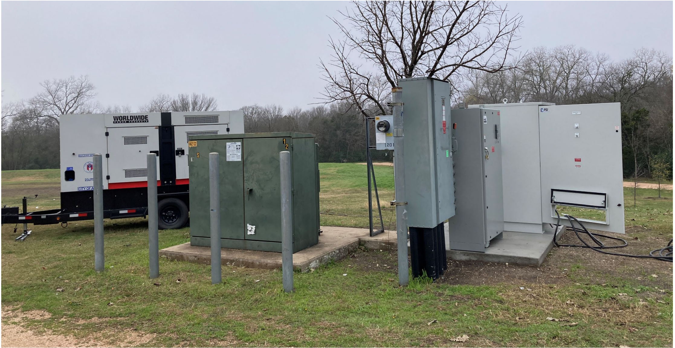
Installed Transfer Switch and Docking Station at Gus Garcia Recreation Center
