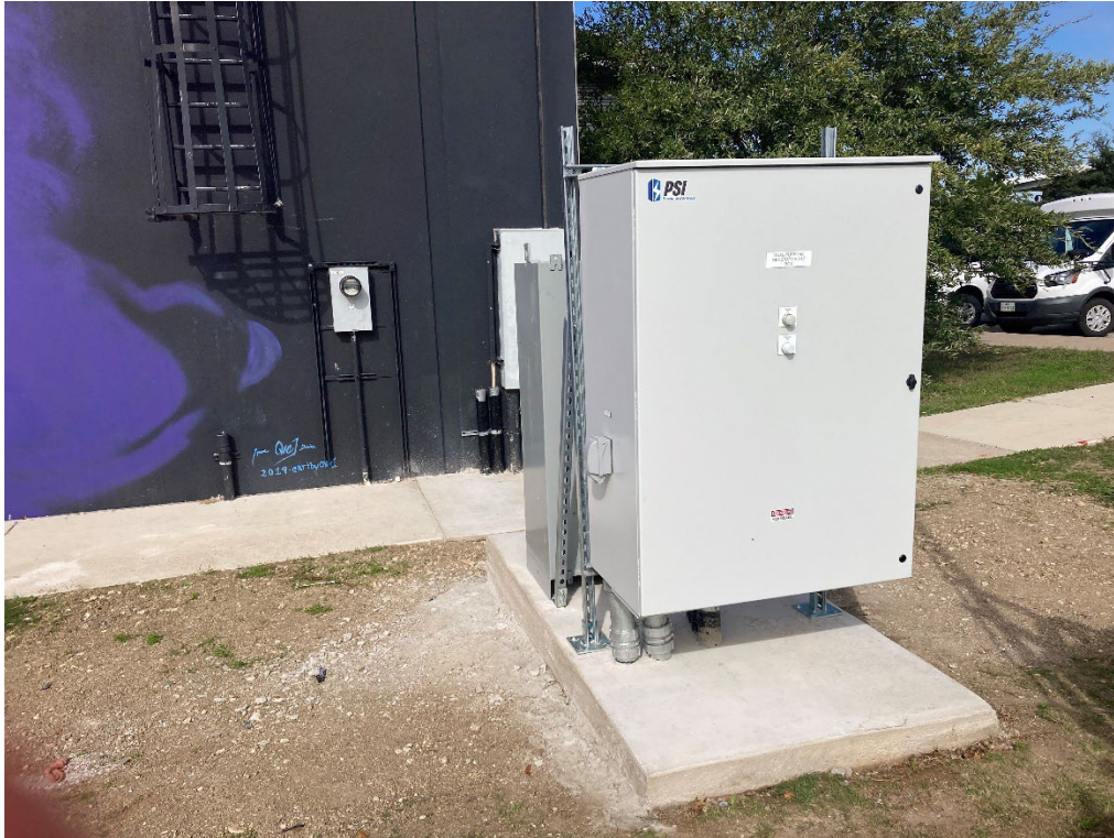
New docking station for redundant power at Turner Roberts Multipurpose Gymnasium.
