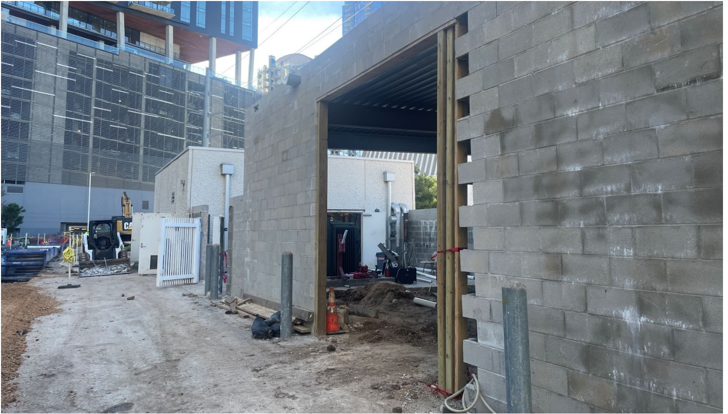
Central Utility Plant: Temporary sawtooth opening for large equipment to be placed in room.
