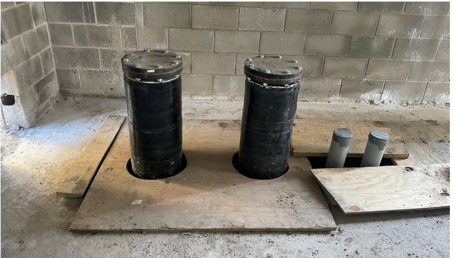
Central Utility Plant: Austin Energy chilled water lines stubbed up and ready to be connected to the heat exchanger.
