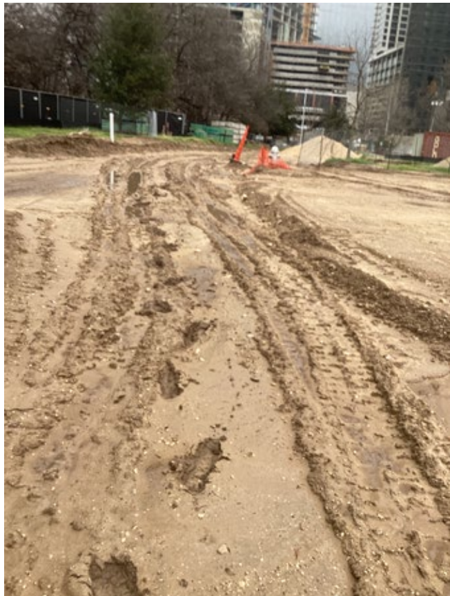
Site: Heavy equipment unable work on future fire lane.
