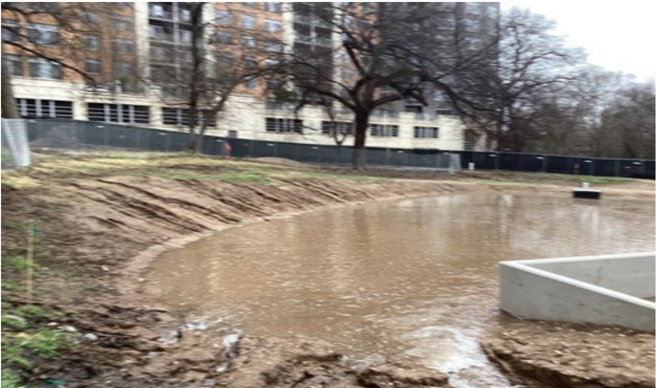
Site: Water Quality Pond filled from rain event. Water must be pumped out to continue work.
