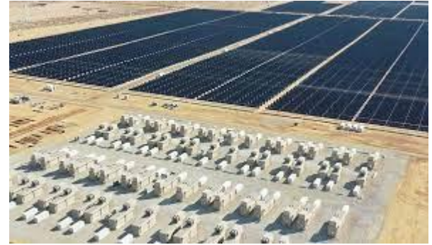
Solar Plus Storage in California's Mojave Desert (875 megawatts from solar along with 3,287 megawatt-hours of energy storage)
