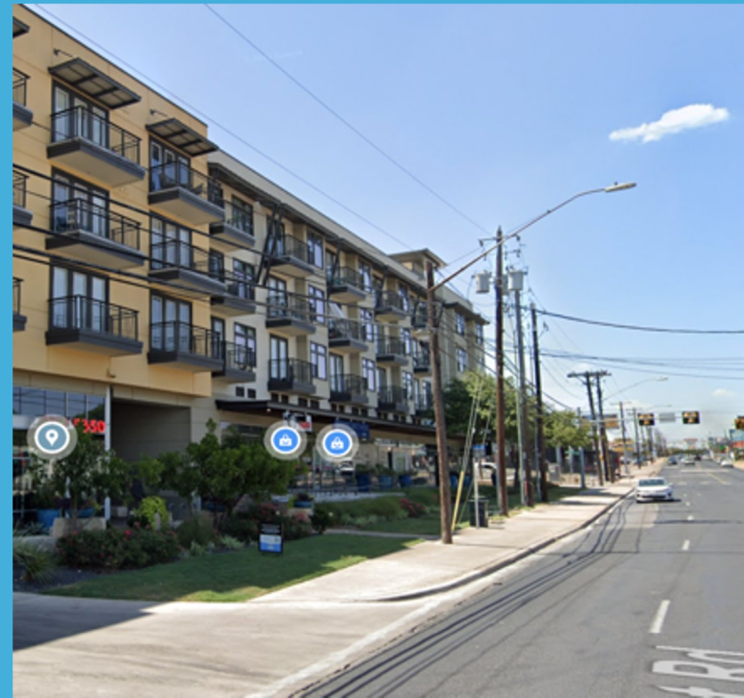
Examples of overhead electric lines that precluded shade trees in the ROW
