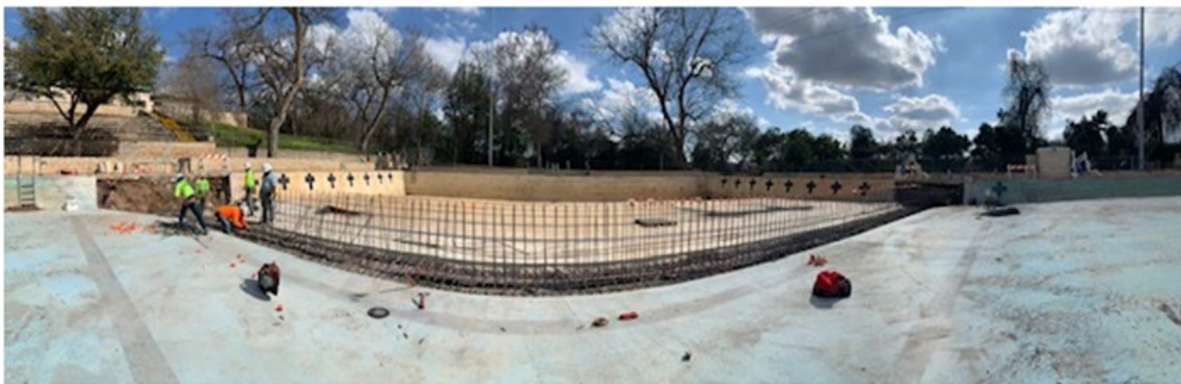
Steel reinforcements have been installed in the keyway for the concrete forms
