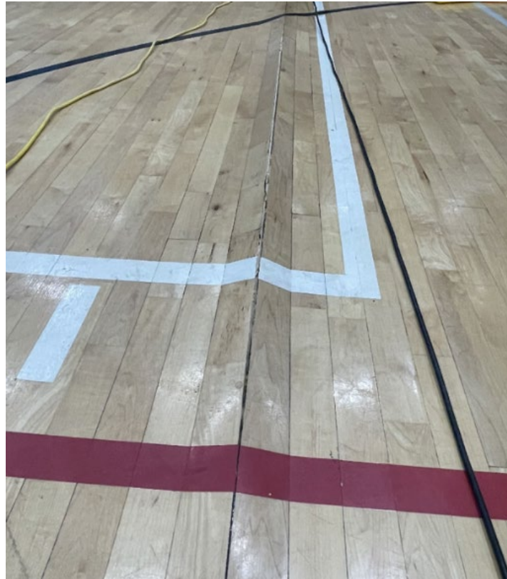
Gus Garcia damaged wood gym floor
