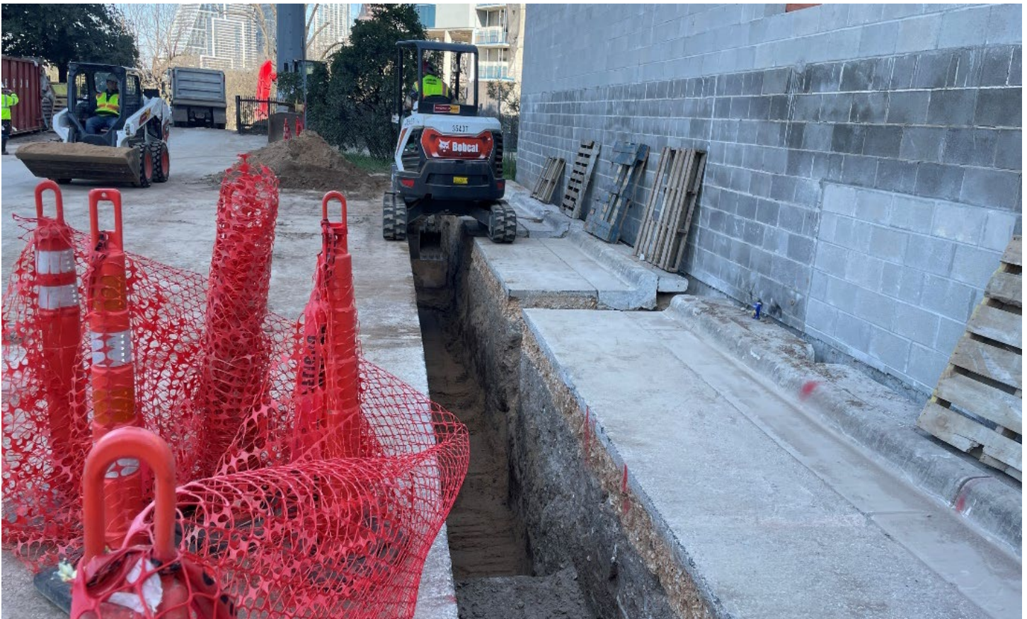
Central Utility Plant: View of trench for wastewater line.
