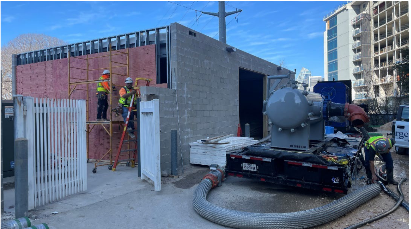
Central Utility Plant: Installation of plywood sheathing to enclose the mechanical room and pipe flushing equipment to remove dirt and contaminants from the new chilled water lines.
