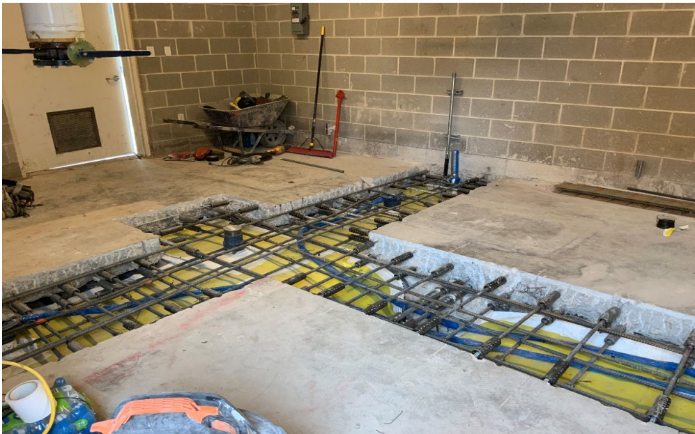
Central Utility Plant – Boiler room ready for concrete pour-back.
