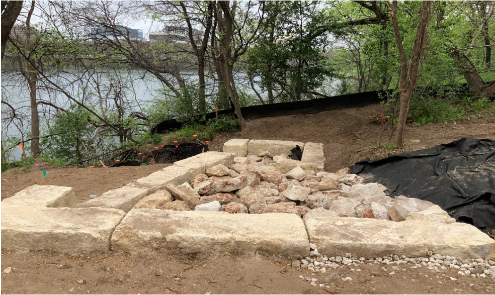
Lady Bird Lake Outfall: Outlet and riprap installed.
