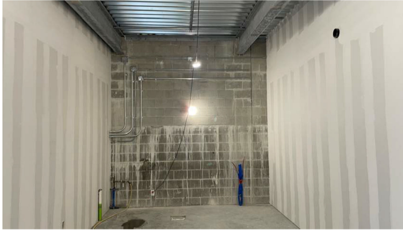
Central Utility Plant: Pump Room framed, taped, and floated drywall installed.
