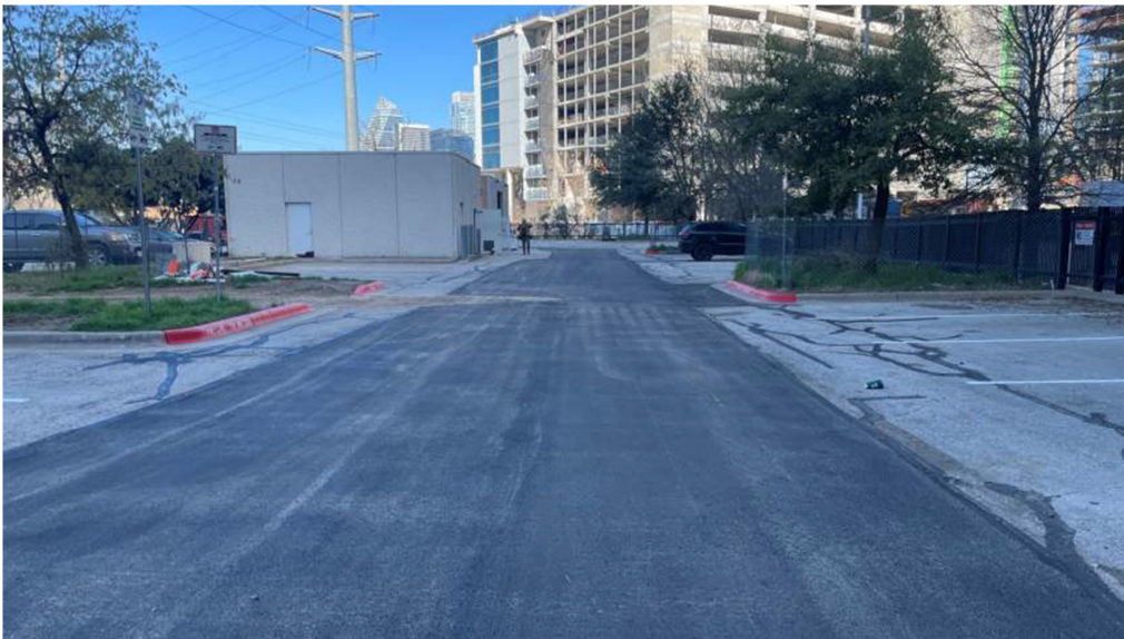
Parking Lot: View of asphalt patching and striping by Austin Energy after chilled water lines were installed.
