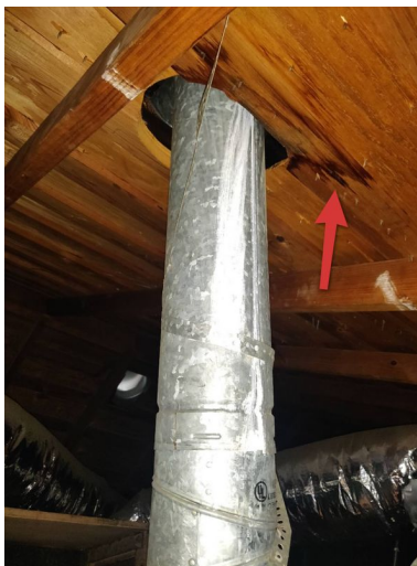
Attic 1 - previous water leaks.
