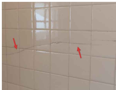
Bathroom - tile crack.
