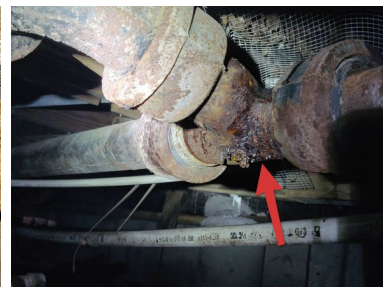
Crawlspace, cast iron sewer/drain line - leak.
