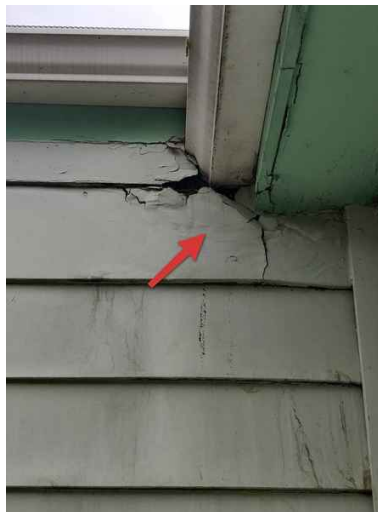
Left side - water damage.
