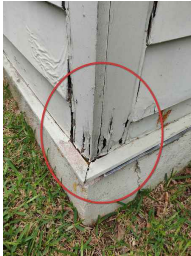
Left side - water damage.
