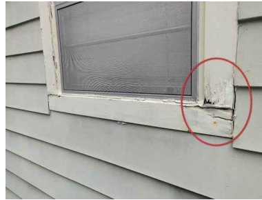
Right side - water damage.
