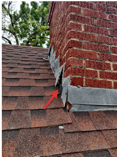
Chimney flashing - loose.
