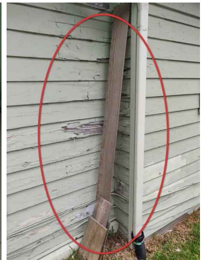
Left side - deteriorated siding.
