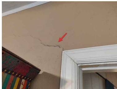
Living room - drywall crack.
