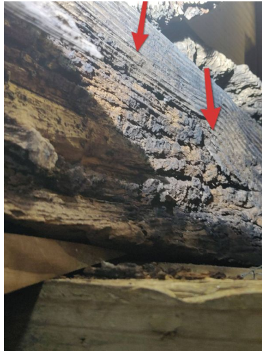
Beam - termite damage.
