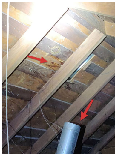
Attic 1 - previous water leaks and range hood exhaust vent.
