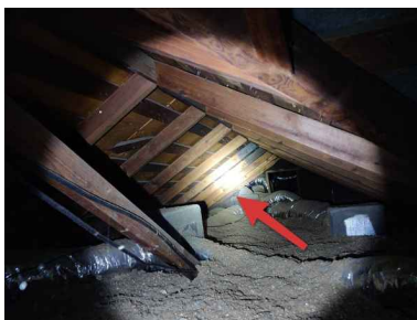
Attic 2 - missing purlin brazing.
