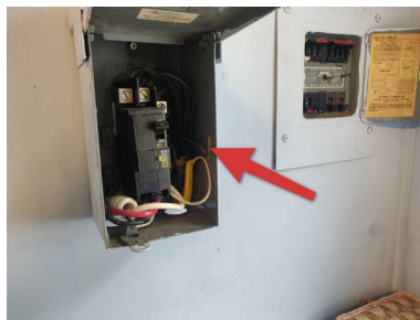
Laundry room, electrical sub-panel - missing cover.
