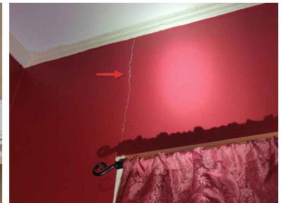
Front right bedroom - drywall crack.
