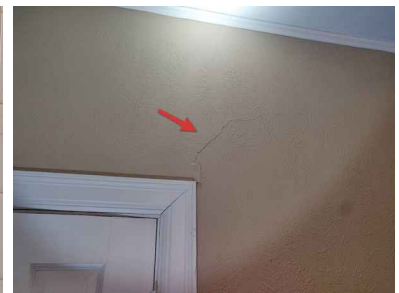
Living room - drywall crack.
