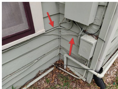
Left side - exposed wiring.
