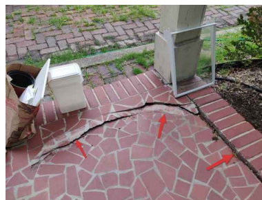
Front porch floor - crack.
