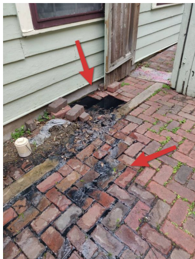
Right side - waste water leak.
