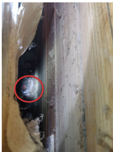
Range gas shut-off valve.
