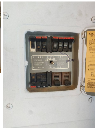
Laundry room, electrical sub-panel - FPE Stab-Lock.
