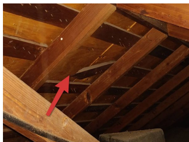
Attic 2, roof decking - damage.
