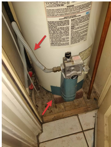
Water heater - missing sediment trap and drain pan.
