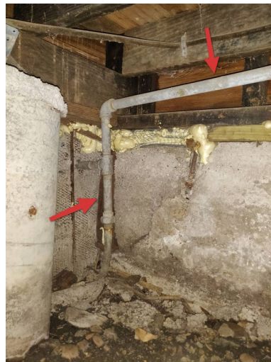
Crawlspace - galvanized water supply line.
