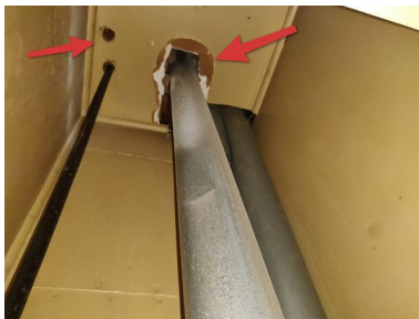
Utility closet ceiling - not properly finished for fire protection.
