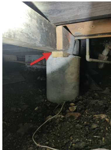
Concrete pier and wood shims.
