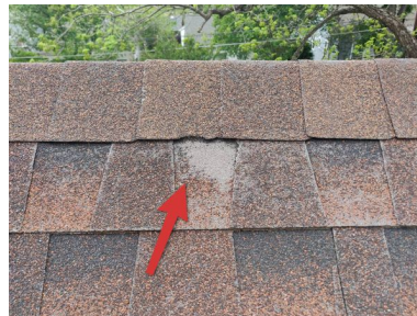
Front - damaged shingle.
