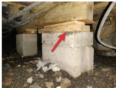
Cinder block pier and wood shims.
