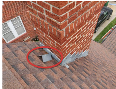
Chimney - loose flashing.
