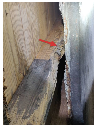
Wall stud - termite damage.
