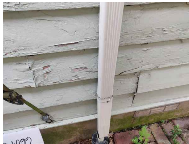
Right side - deteriorated siding.
