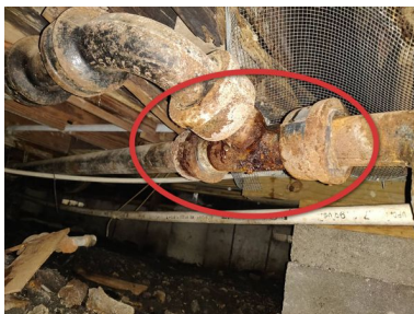
Crawlspace, cast iron sewer/drain line - leak.
