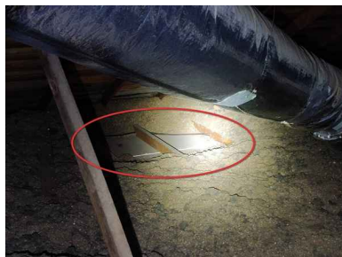
Attic 1 - missing insulation.
