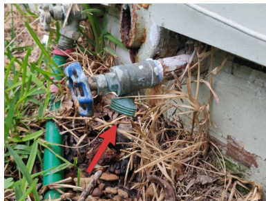
Left side - missing vacuum breaker.
