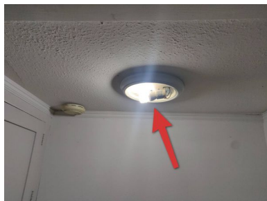
Hallway - missing guard cover.
