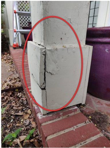
Front porch column - water damage.
