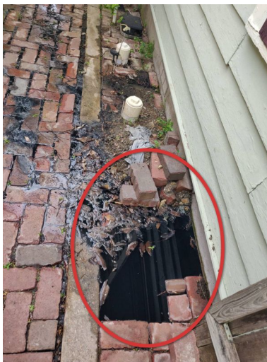
Right side, waste water leak - strong odor.
