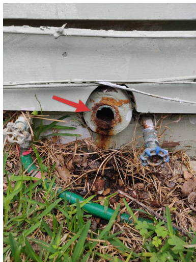
Left side, cast iron cleanout - missing cap.
