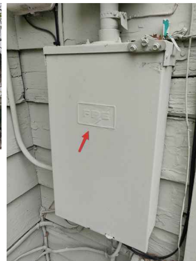
Main electrical panel - Federal Pacific Electric (FPE).
