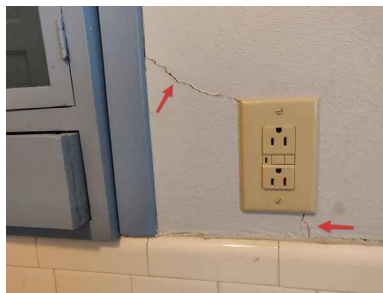
Bathroom - drywall crack.
