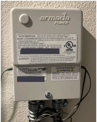
Multifamily Smart Home: Armada Power Water Heater Controller & Ecobee Thermostat
