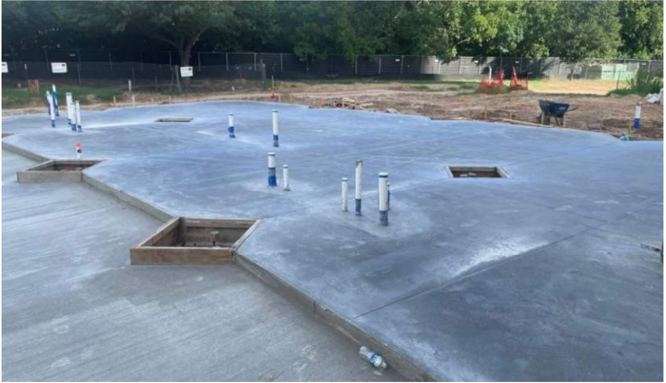
North Building Addition: Foundation slab.
