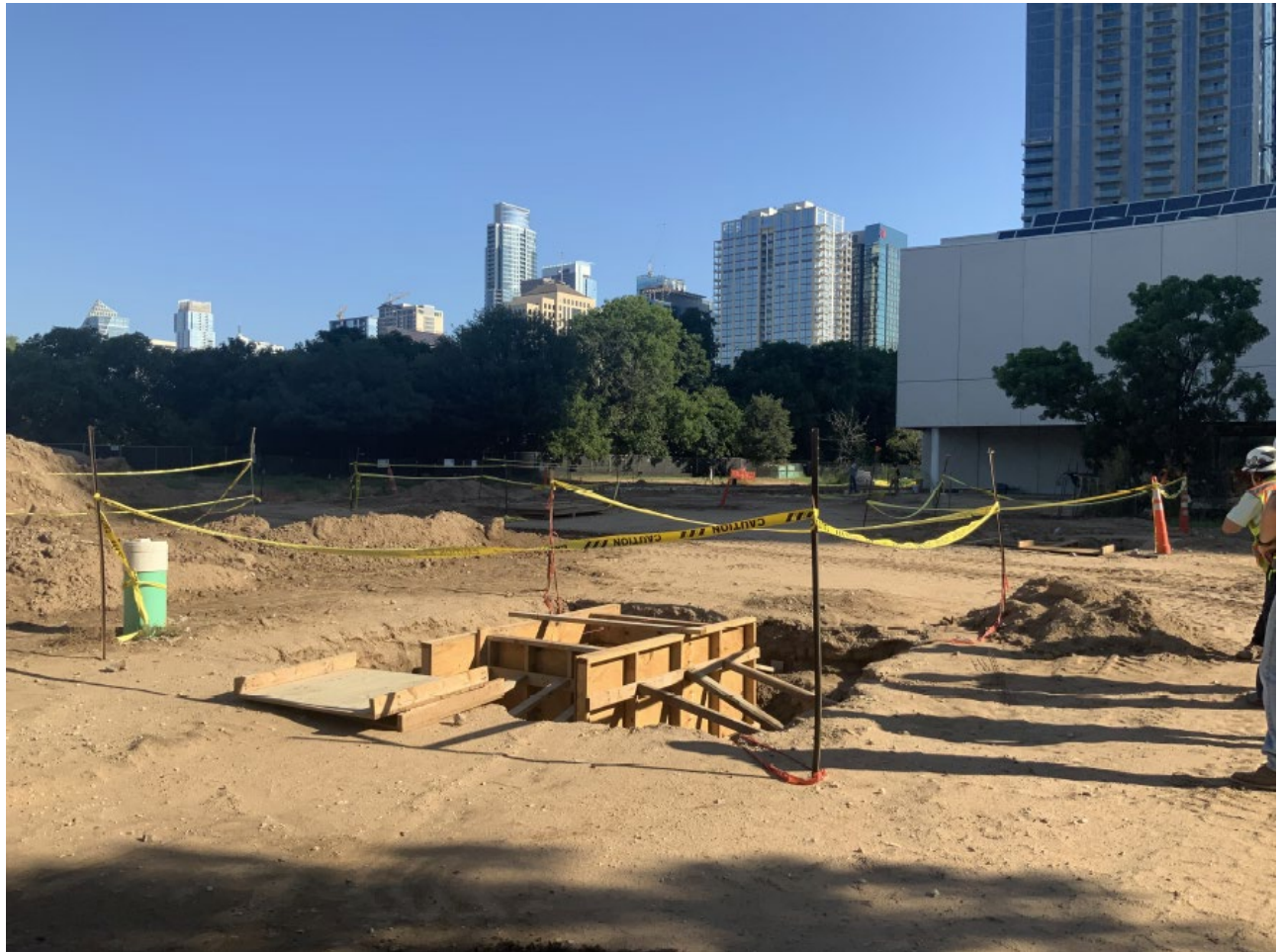
Zocalo: One of four foundation piers for the shade structure.
