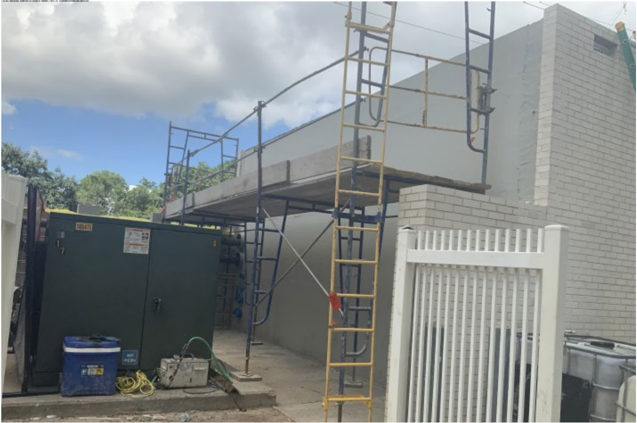
Central Utility Plant (CUP): Stucco wall finish application while in progress.
