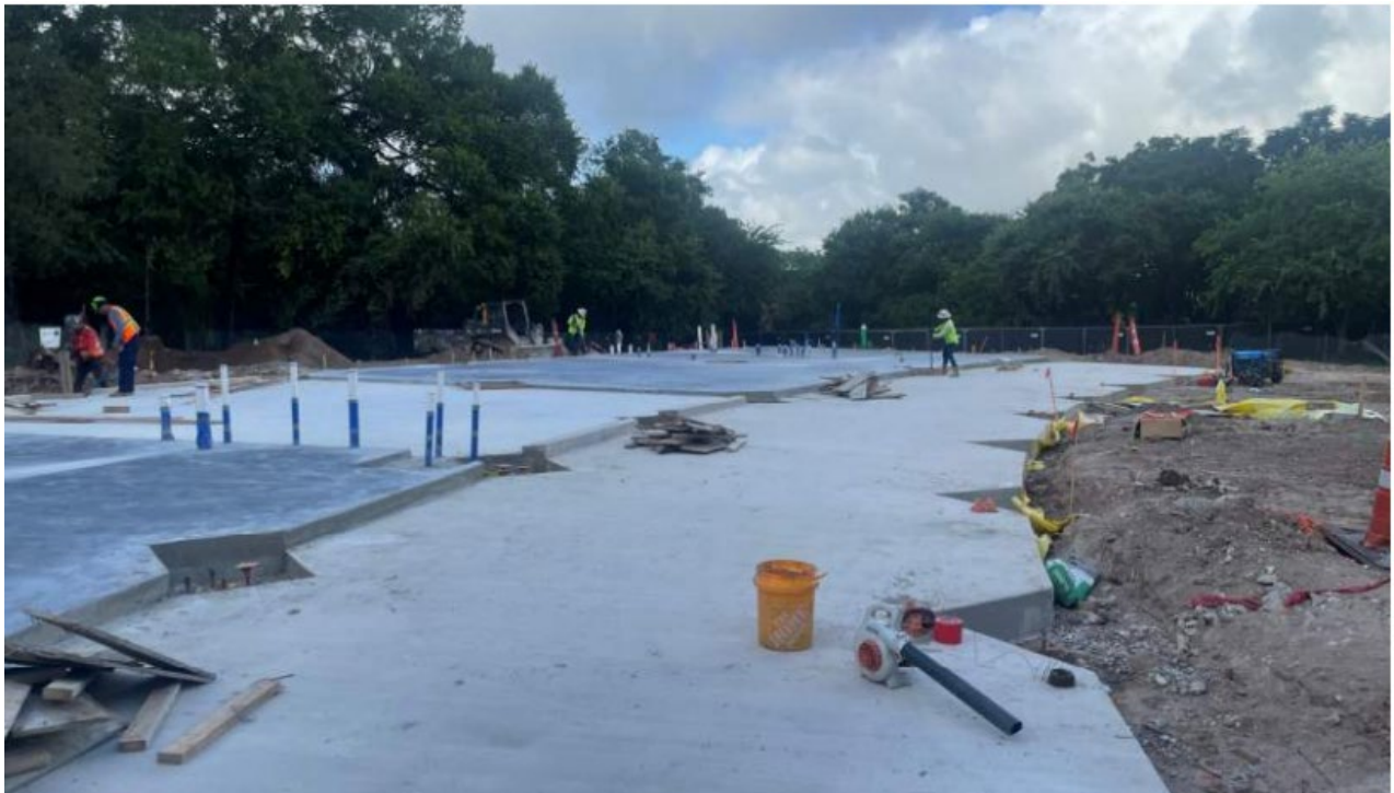
South Building Addition: Foundation slab.
