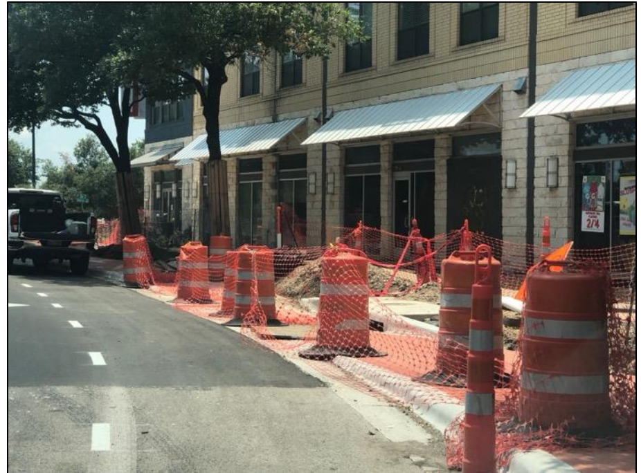
The Aldrich/Mueller roundabout nearing completion
