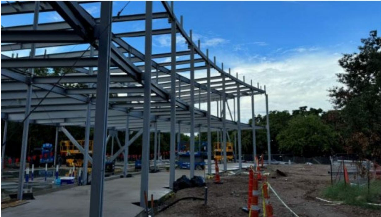
South Building Addition: Steel erection in progress.
