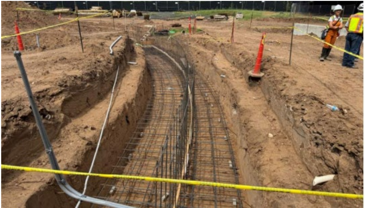
Zocalo: Excavation and rebar installation in preparation for the retaining wall.
