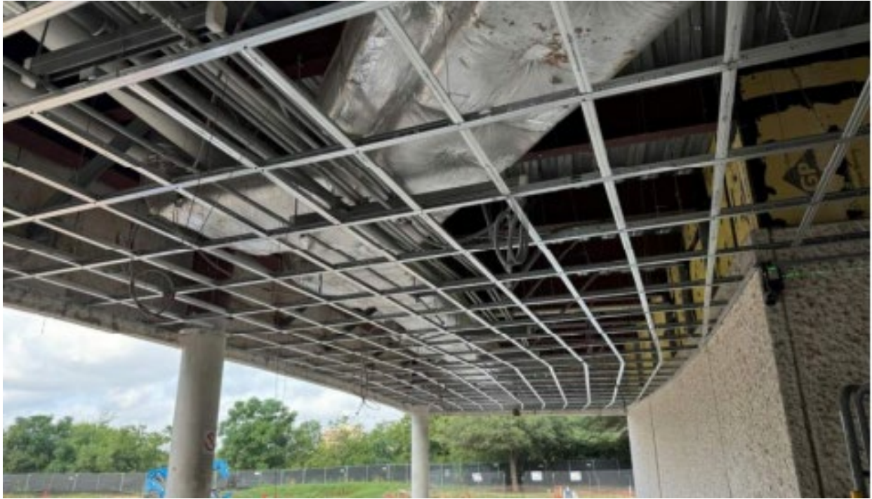
Building: Framing for exterior replacement soffit or ceiling complete.
