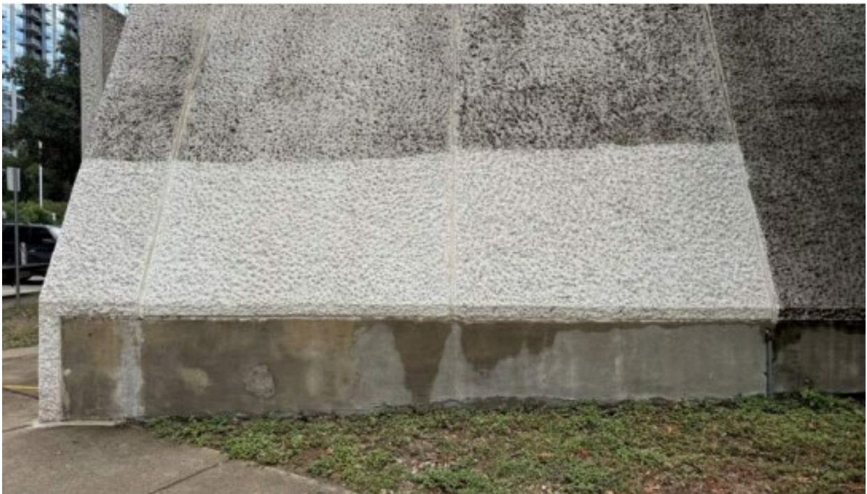
Building: Trial cleaning method of the building exterior.
