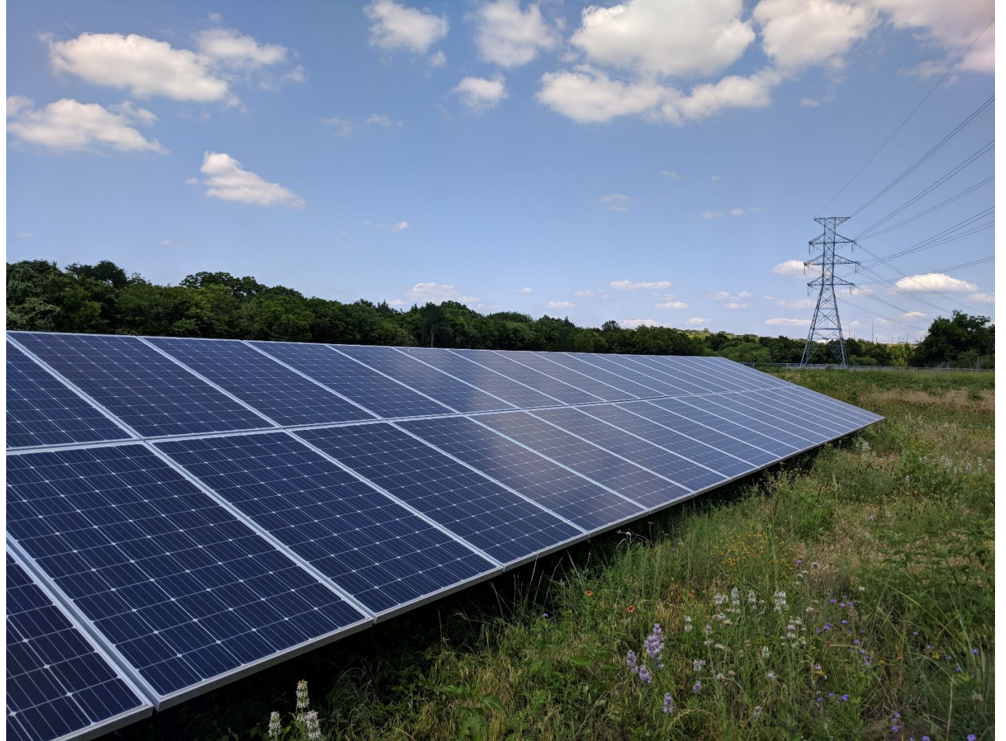
La Loma Community Solar Farm
