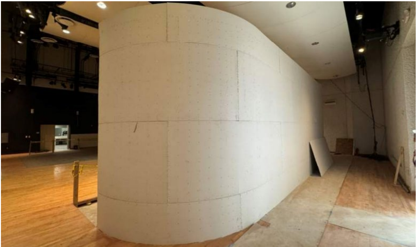
Building: Auditorium new raised control booth.
