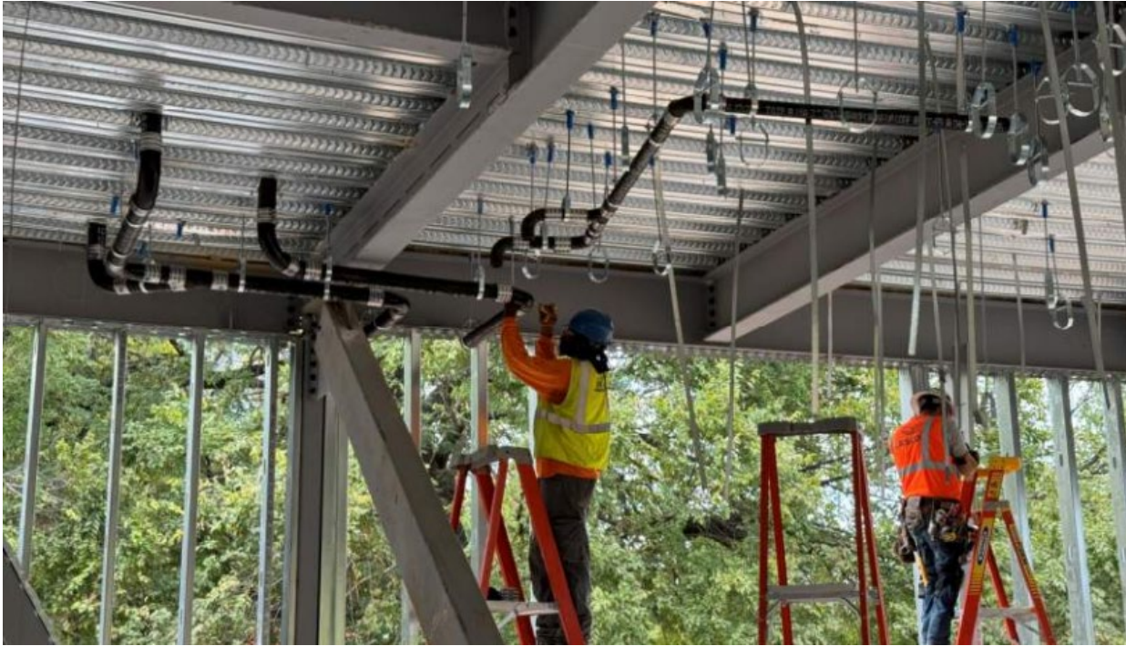
Building: Overhead plumbing being braced.
