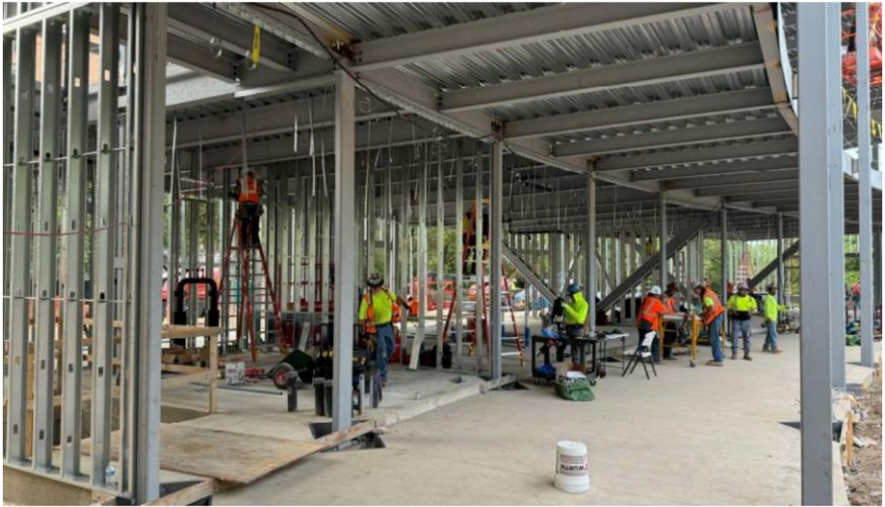
Building: Interior framing in process
