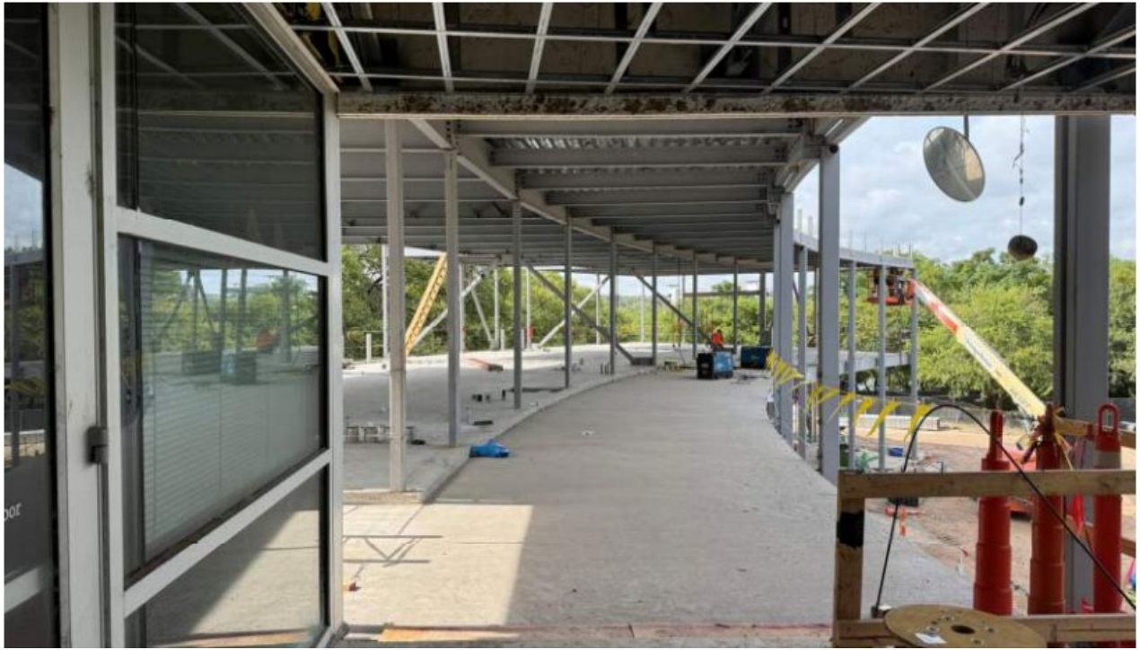
Building: View of level 2 exterior walkway.
