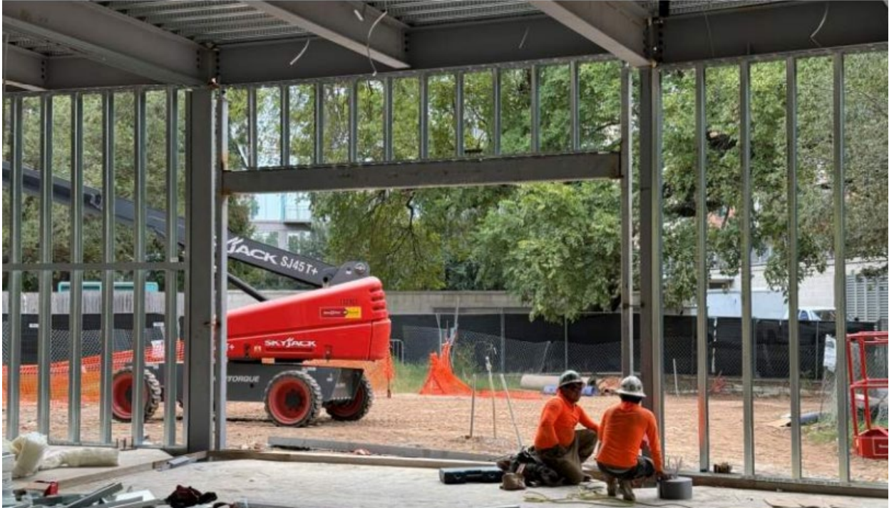
Building: Dance Studio framing in process
