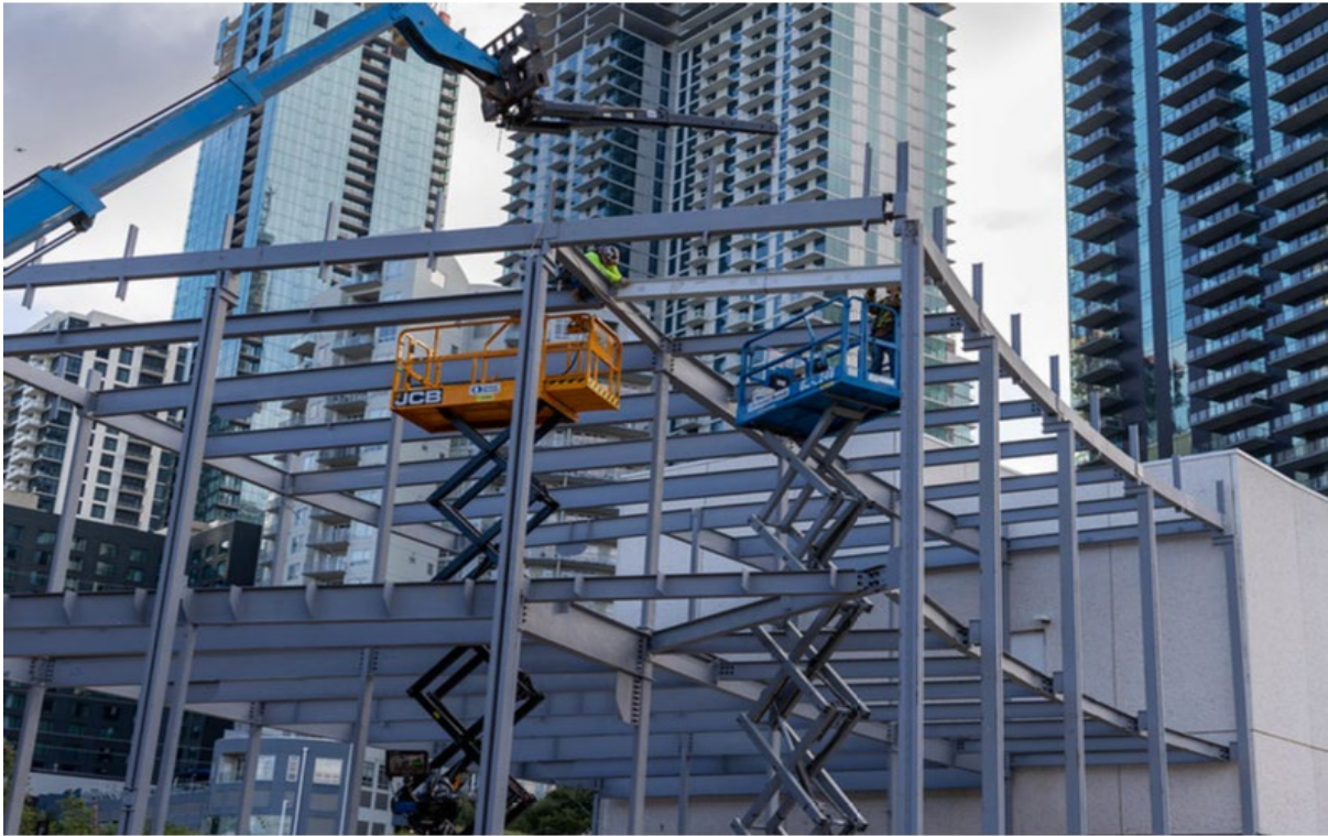
Topping Out: Signed top beam lifted and welded into place.
