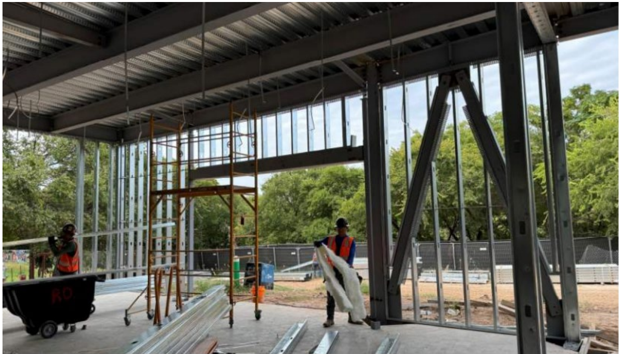
Building: Teaching kitchen framing in progress.
