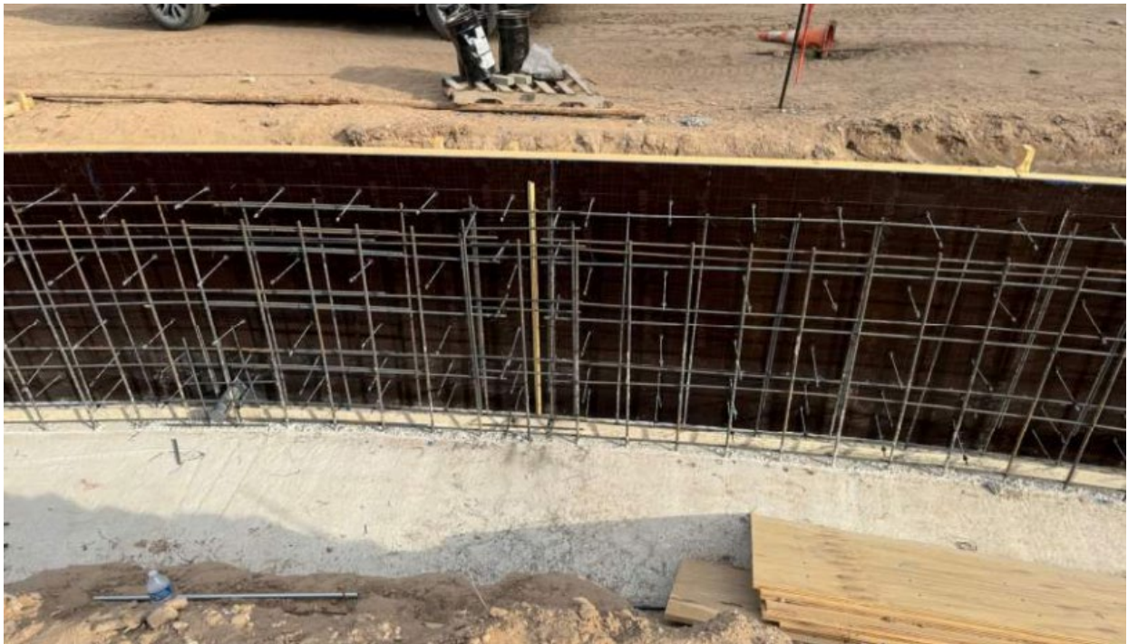
Site: Forms and reinforcement for retaining walls in progress.
