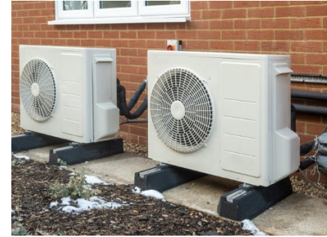
Ductless mini-split: exterior and interior units
