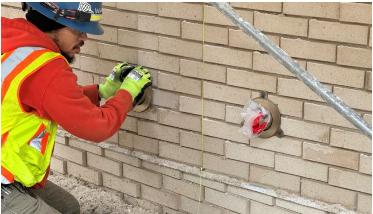
South Addition: Brick work and roof downspouts outlets installation in progress.
