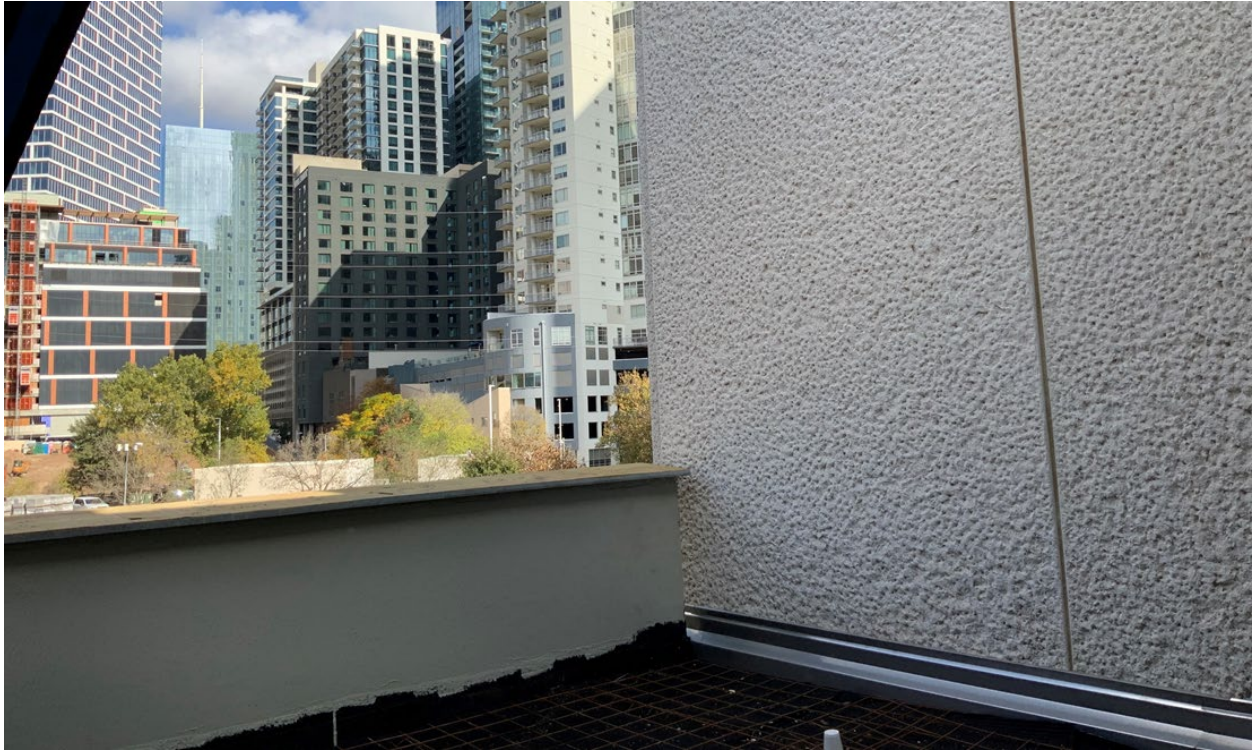
North Addition: Outdoor terrace waterproofing and flashing underway.
