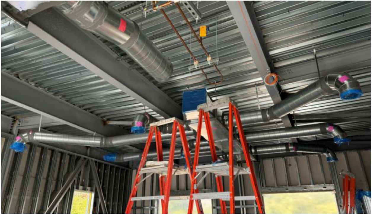
North Addition: Overhead ducts installation of mechanical systems.
