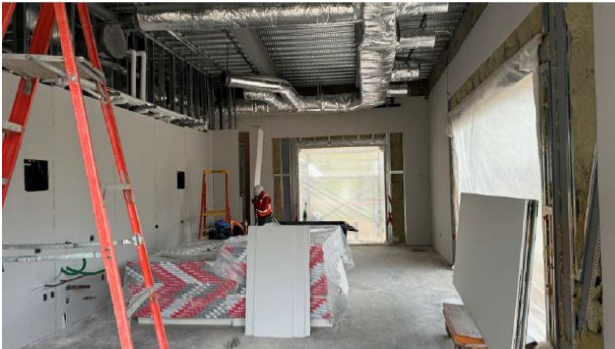
South Addition: Teaching Kitchen receiving drywall and insulation after passing inspection.
