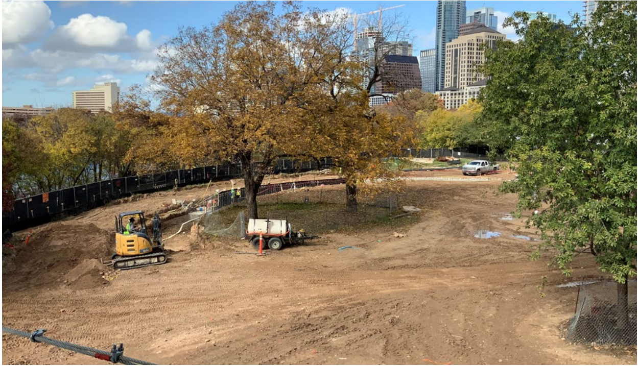
Zocalo: Retaining wall construction in progress.
