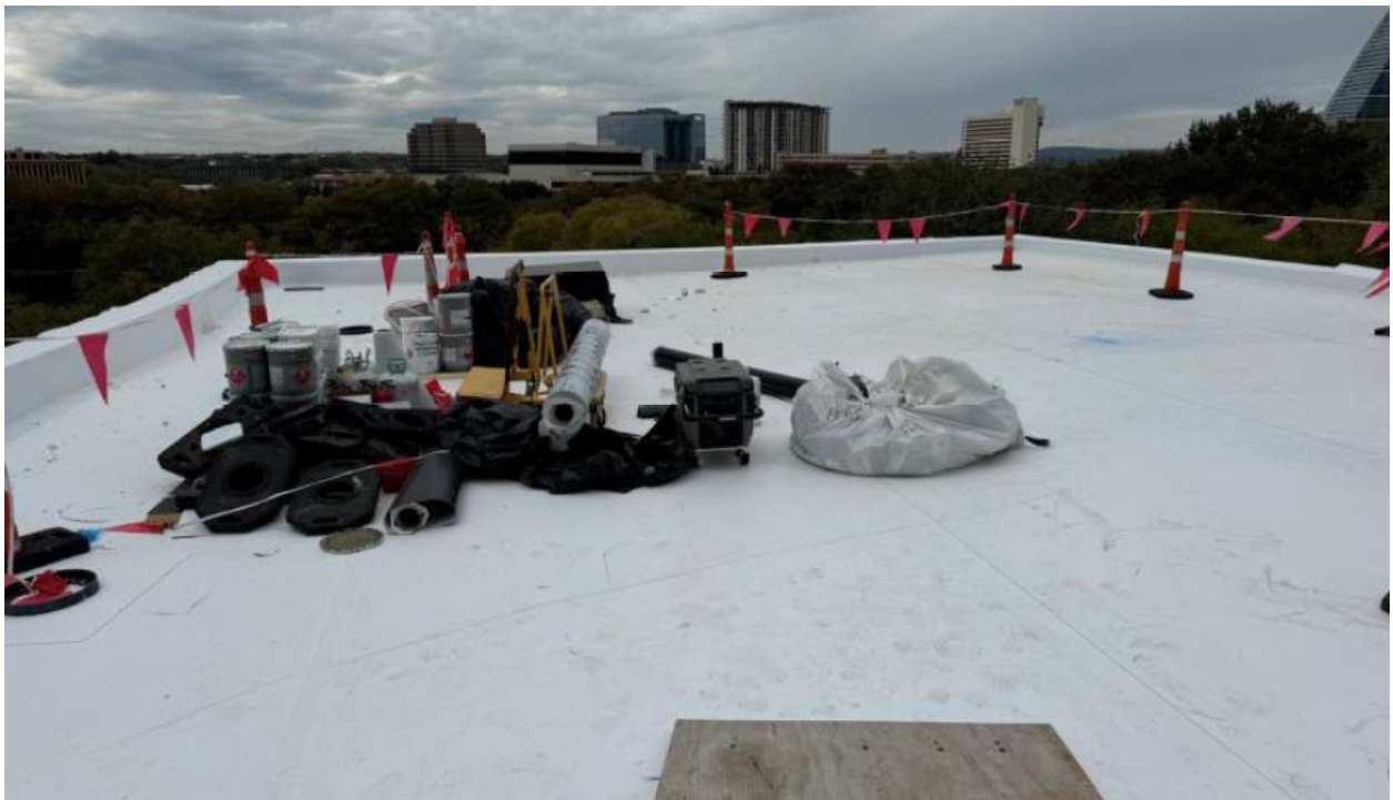
North Addition: View of roofing progress.
