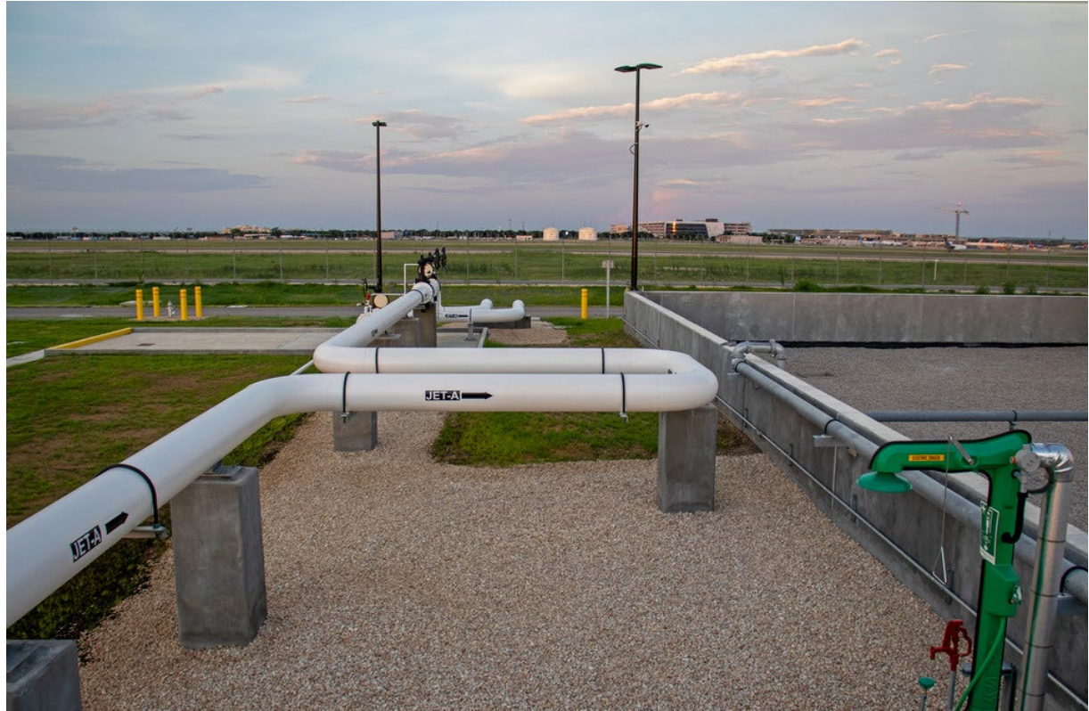
View of transfer pipeline – looking east
