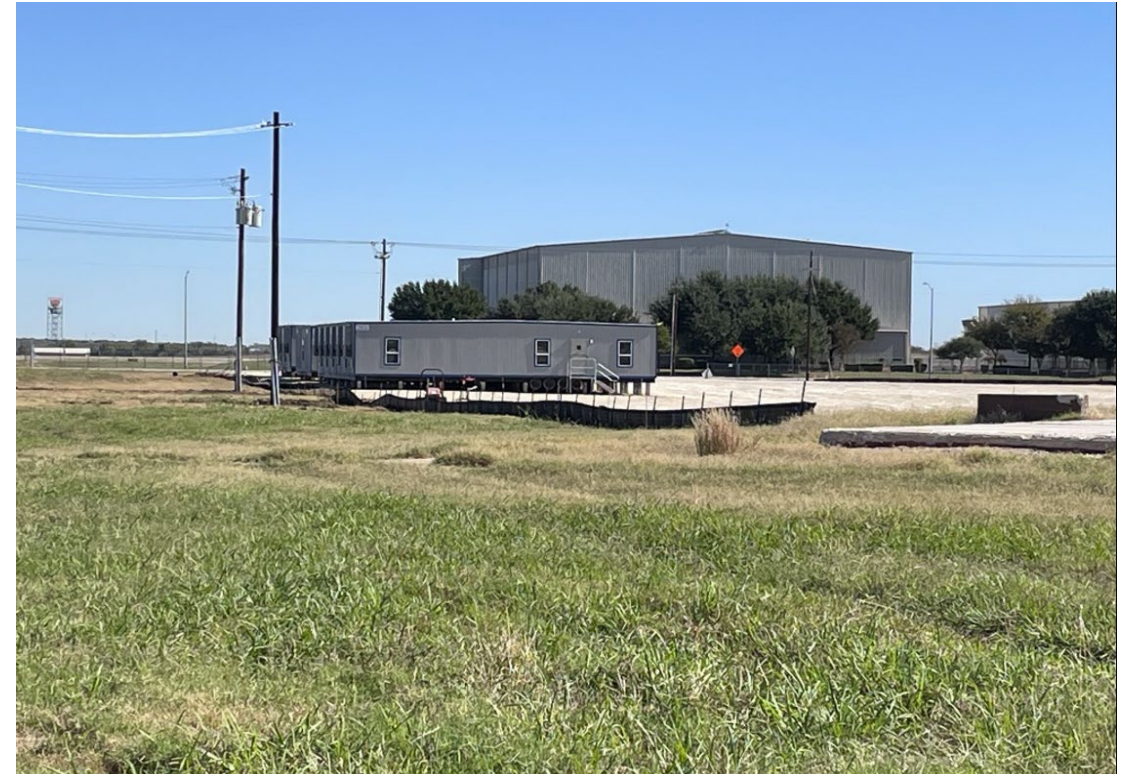
Contractor setting up staging yard
