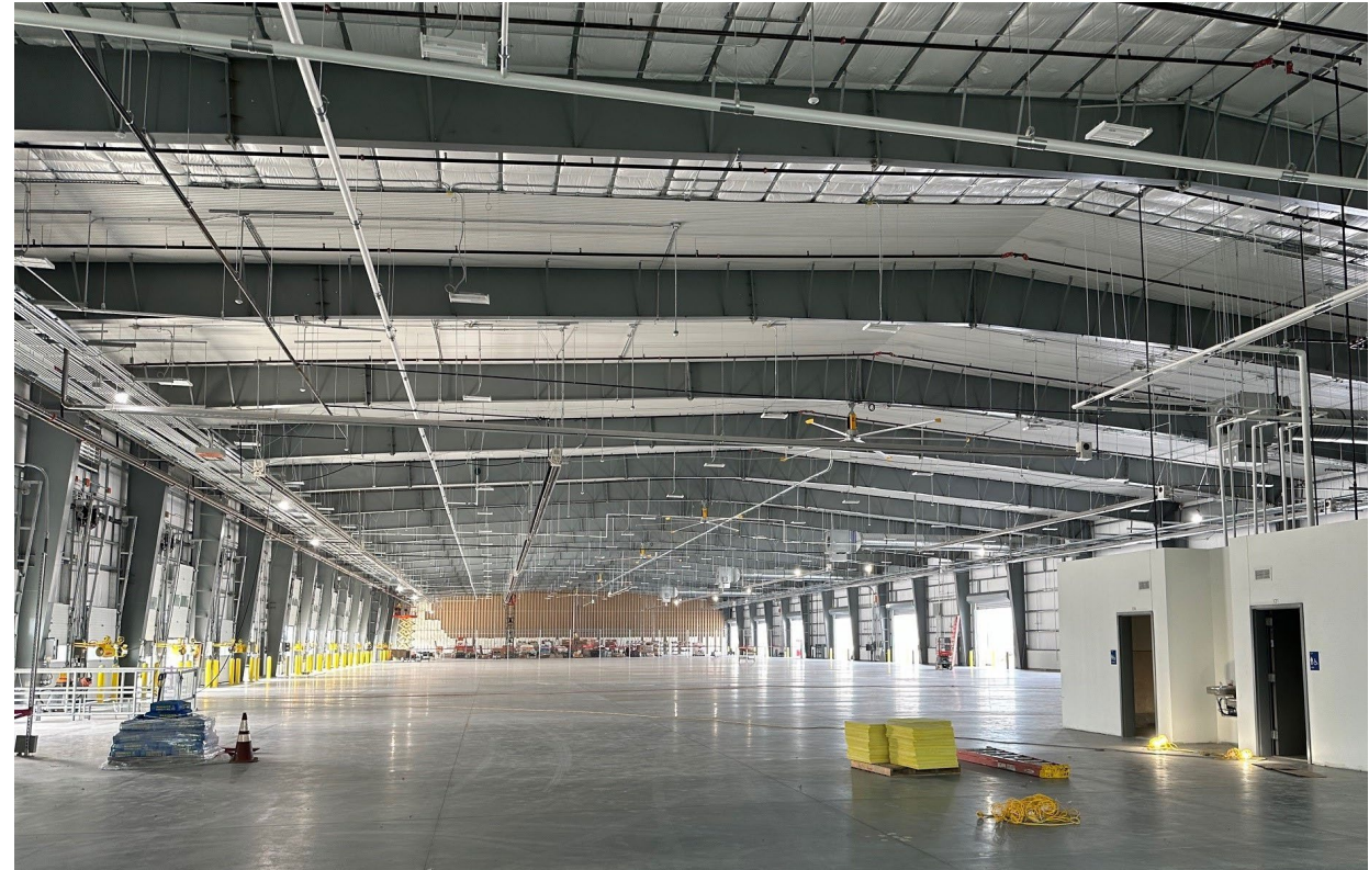
Interior – New East Cargo Building
