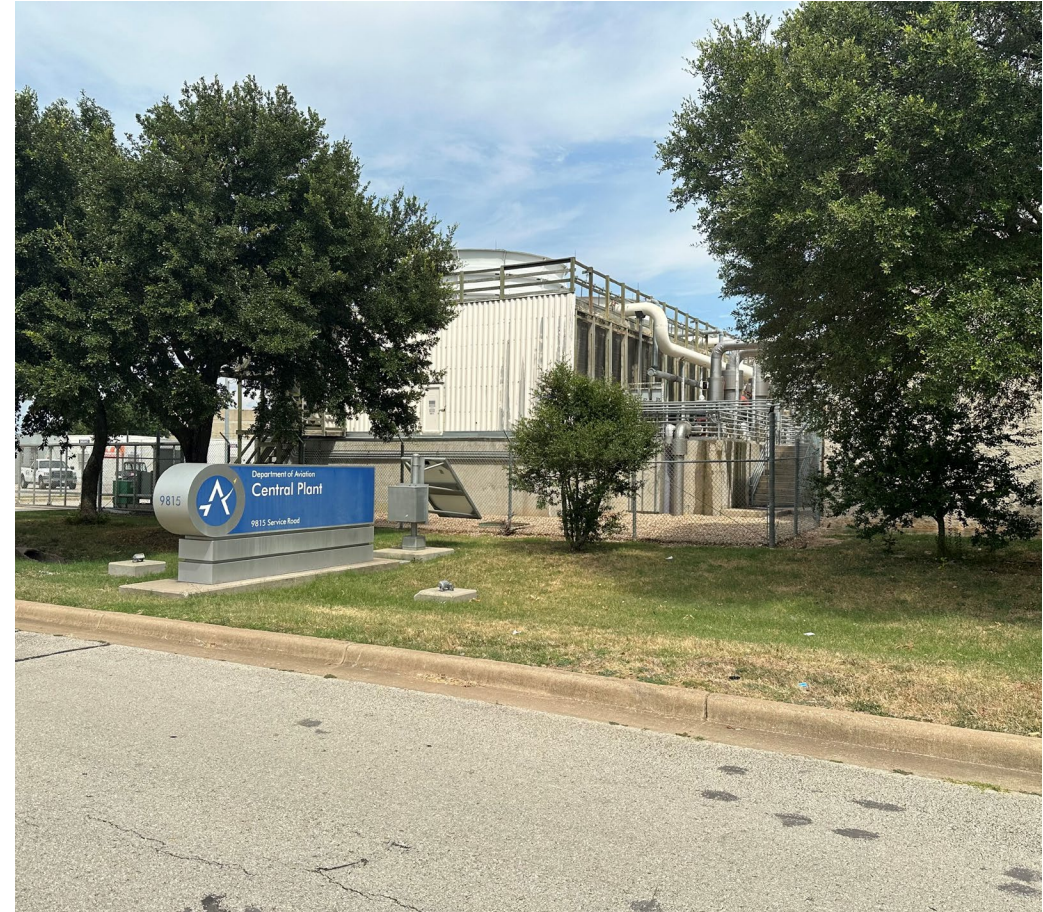
Current Central Utility Plant
