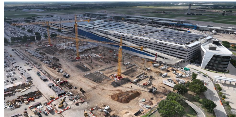
Construction photo showing project progress as of June 30, 2025.
