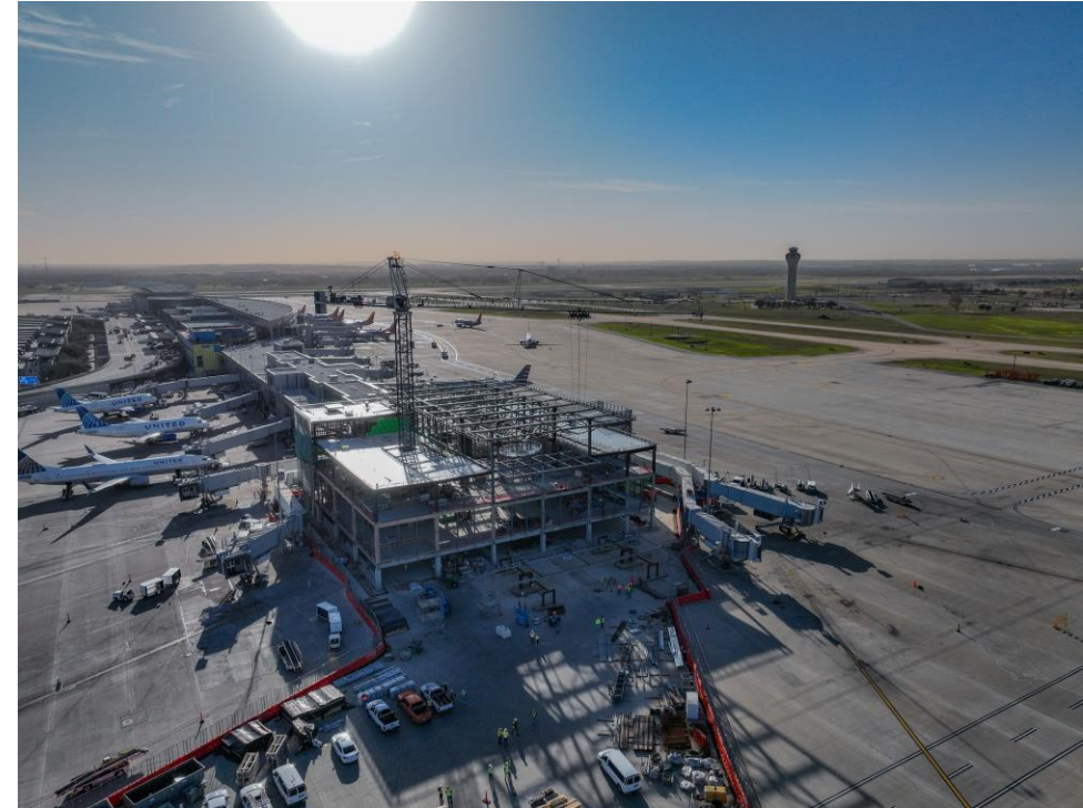
Aerial photo of West Gates under construction.
