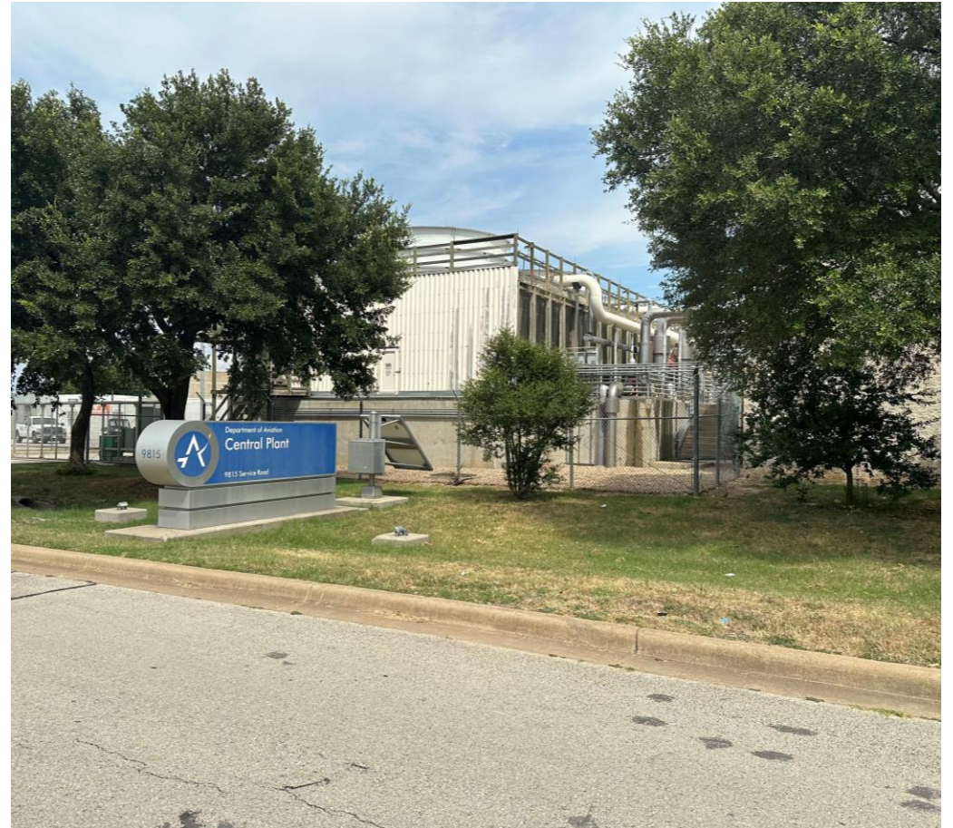
Current Central Utility Plant
