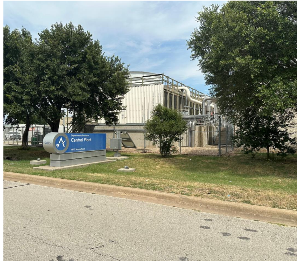
Current Central Utility Plant
