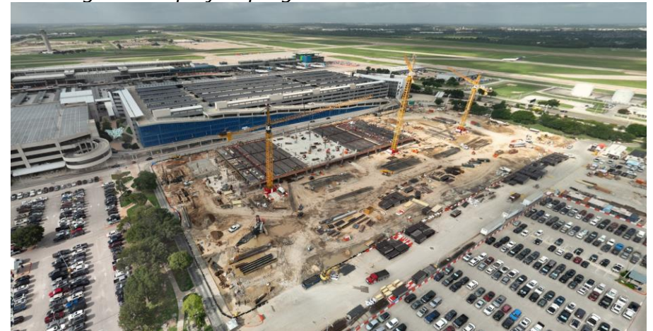
Construction photo showing project progress as of July 14, 2025.
