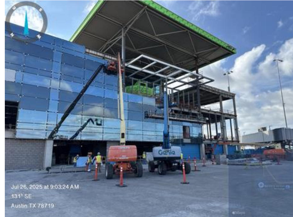
Photo of the West Gate project under construction.
