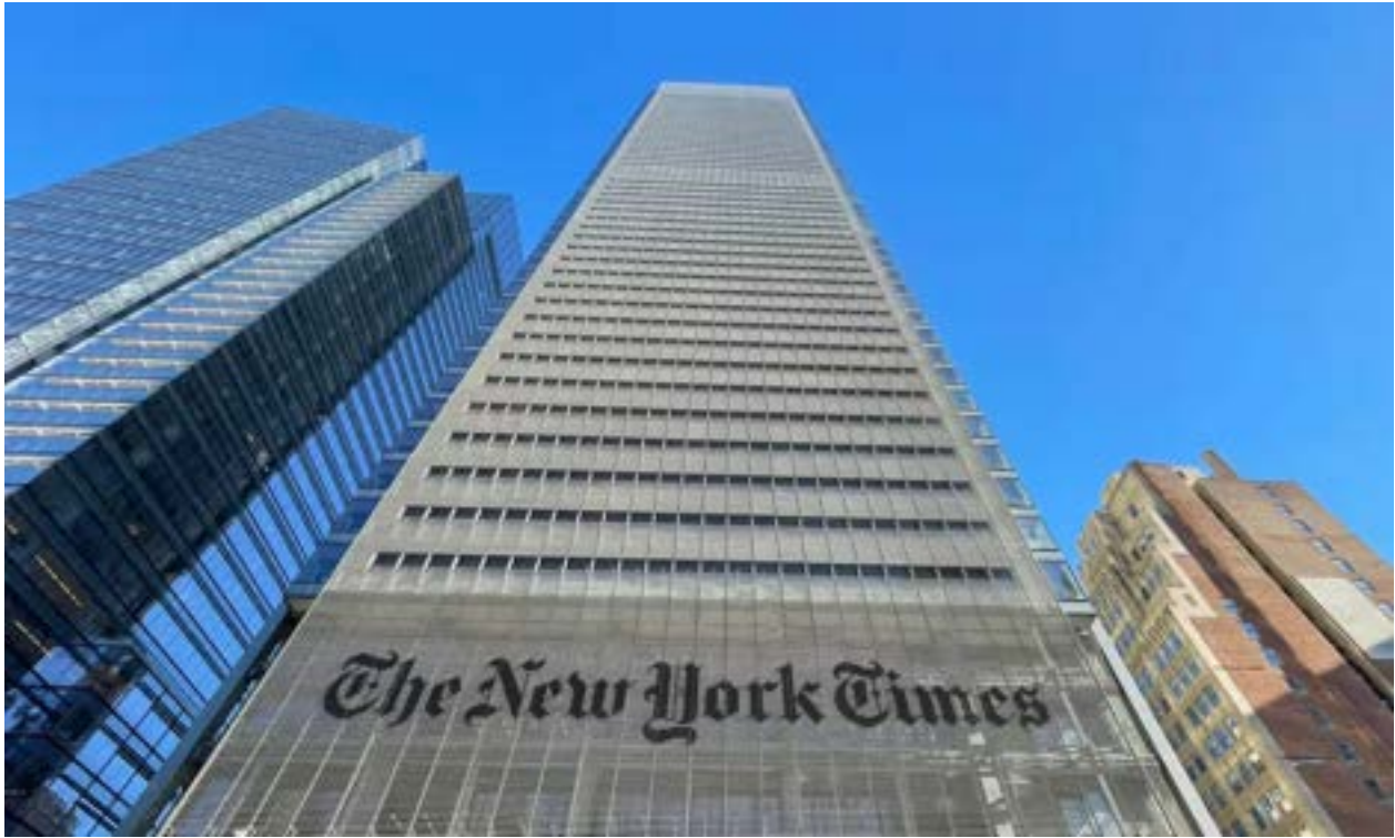
The New York Times building uses fritted glass clad with rods, which make its facade more visible to birds. Photograph: Daniel Slim/AFP/Getty Images
