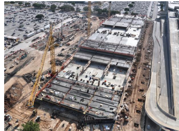
Construction photo showing project progress as of Aug 27, 2025.
