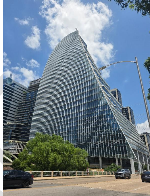
Google Austin building in downtown Austin.
