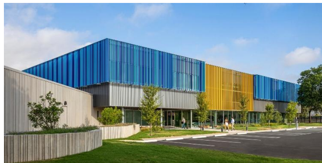
Austin-Bergstrom International Airport (AUS) IT Building. Photo by PAGE
