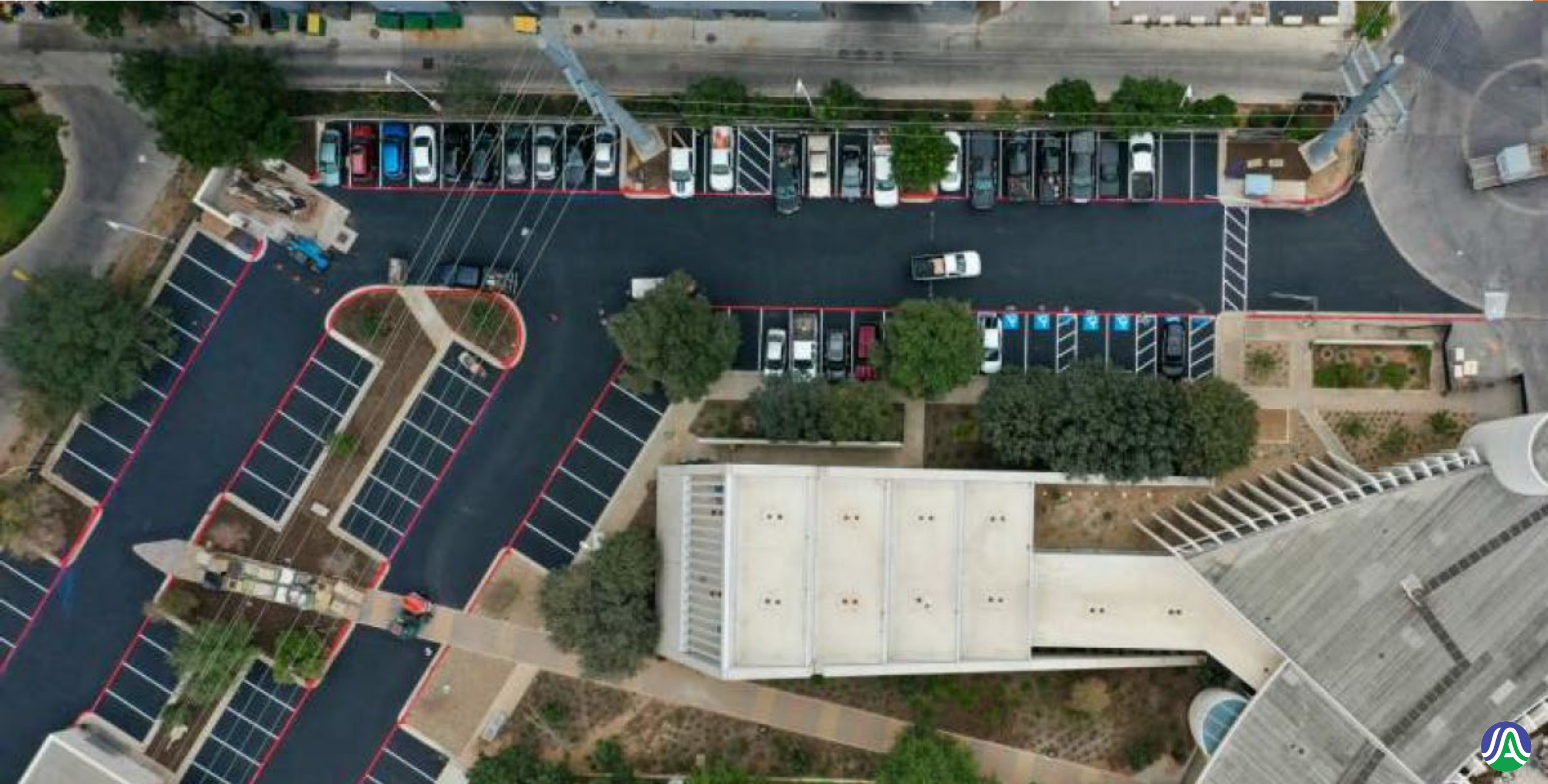
Parking Lot: Seal coat and restriping was completed.
