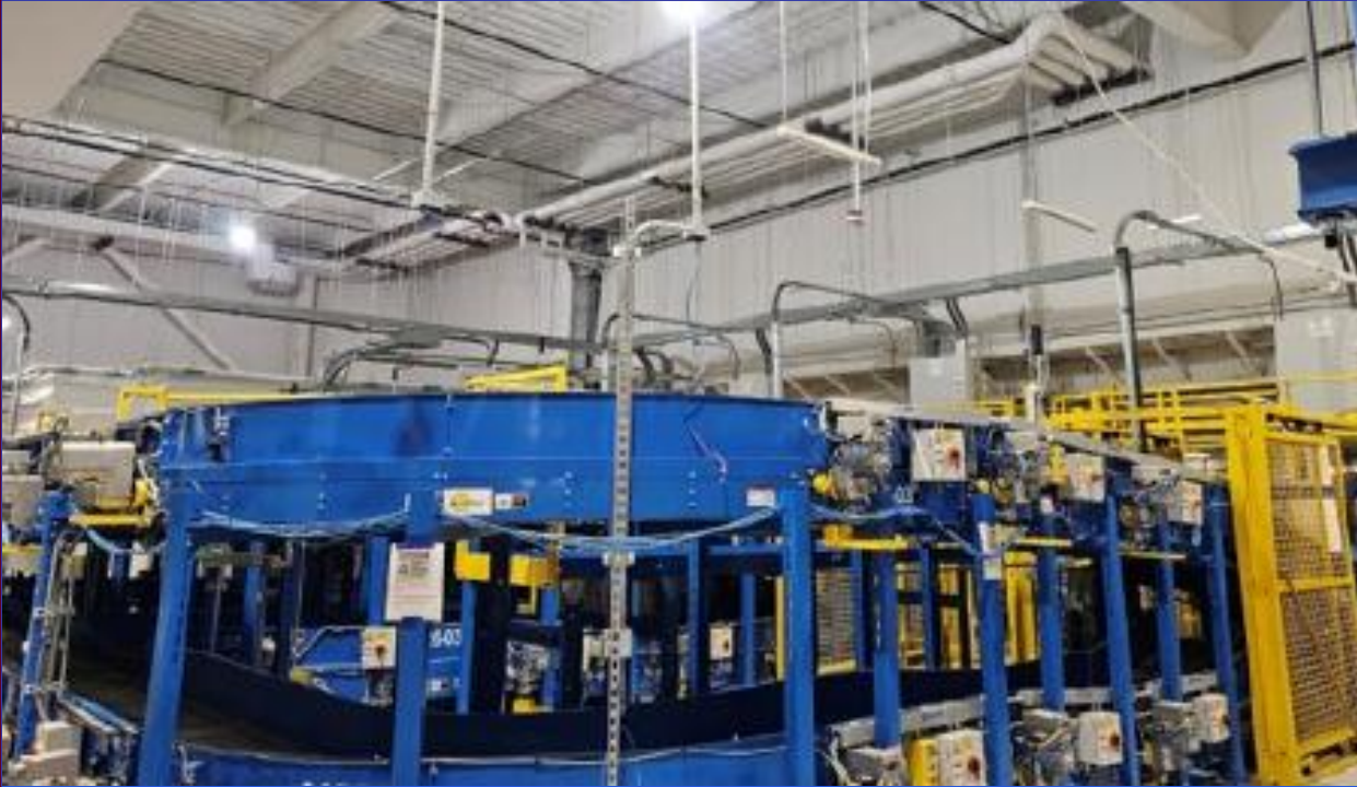
Baggage Handling System testing
