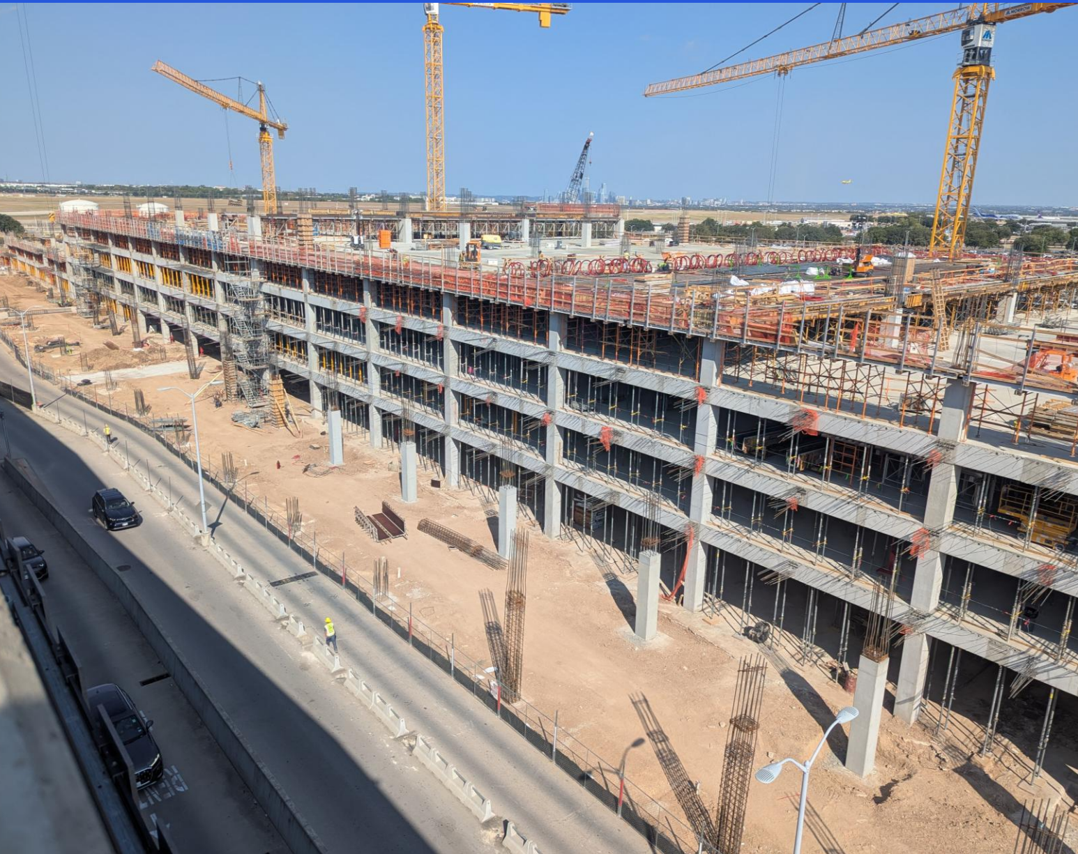
Garage viewed from the south
