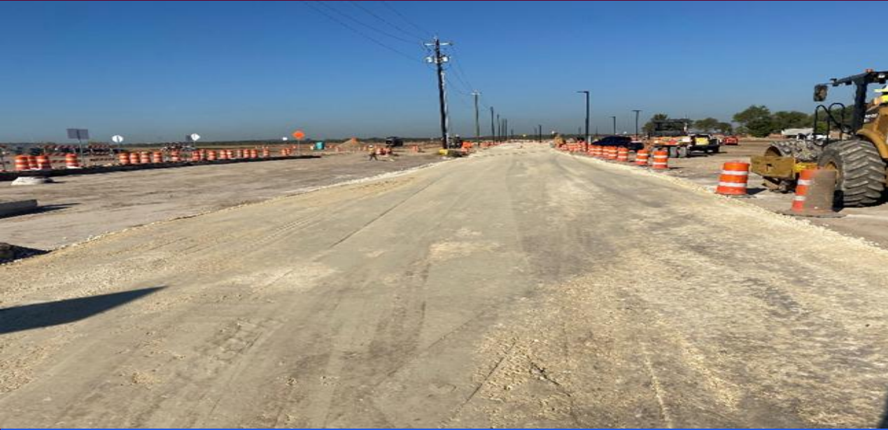
Placement of crushed rock foundation base on Fighter Drive
