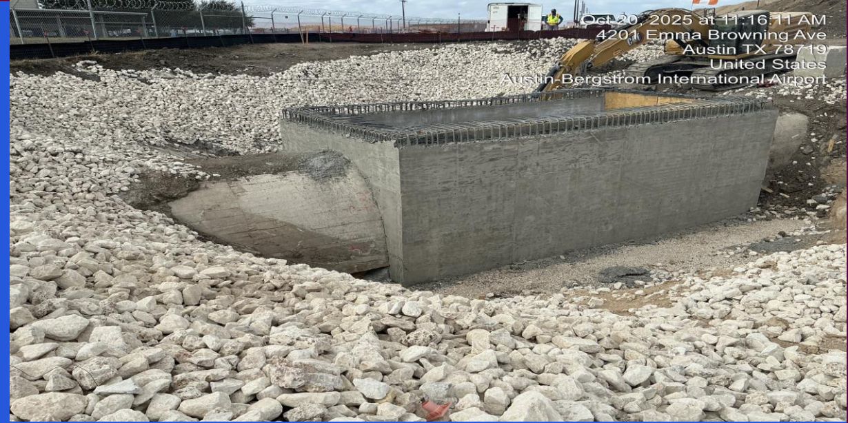
Phase 3 48" reinforced concrete pipe installation
