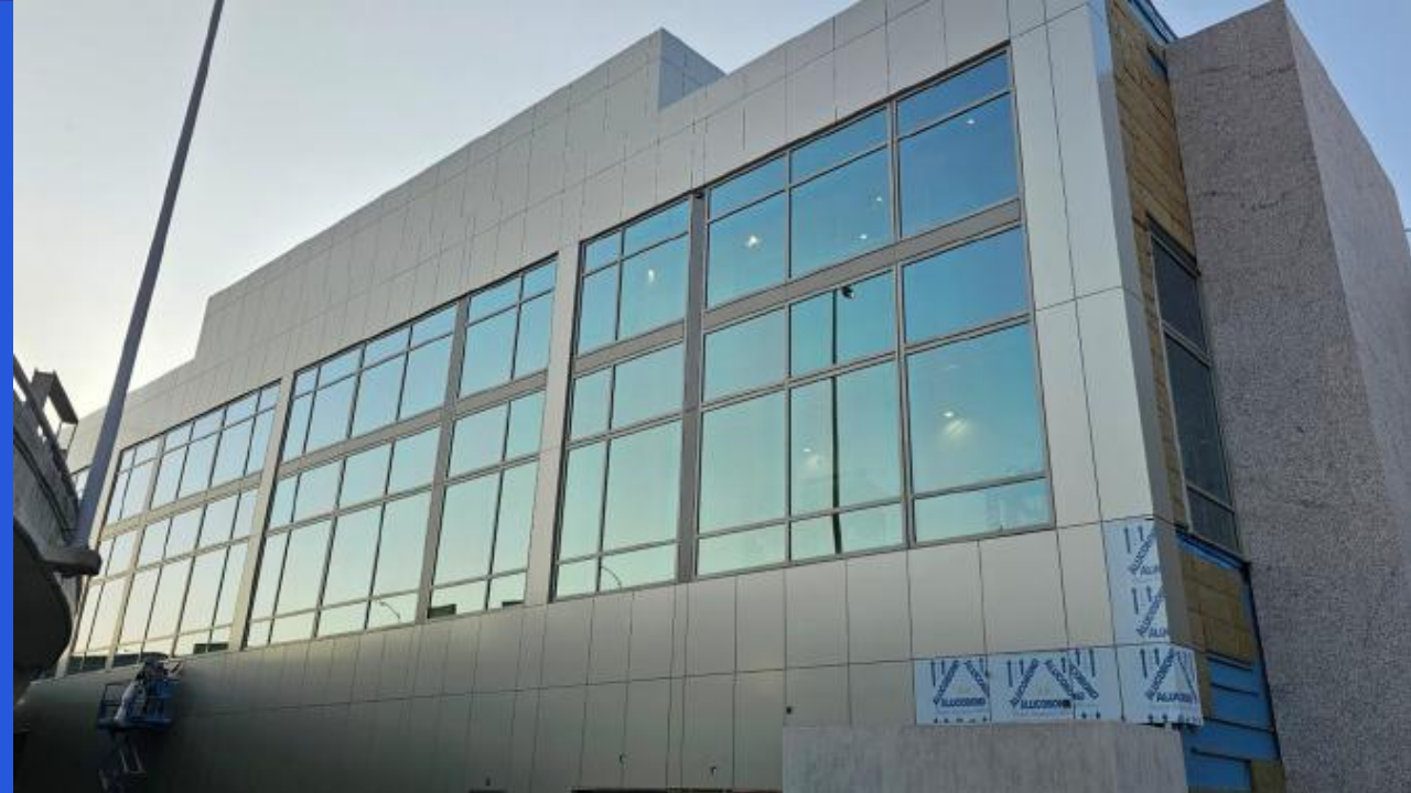
Exterior metal panel installation
