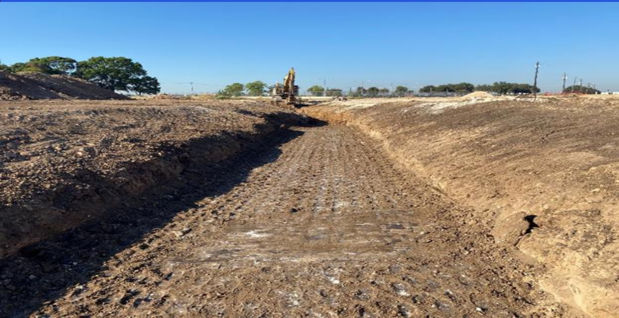
Placement of crushed rock foundation base on Fighter Drive
