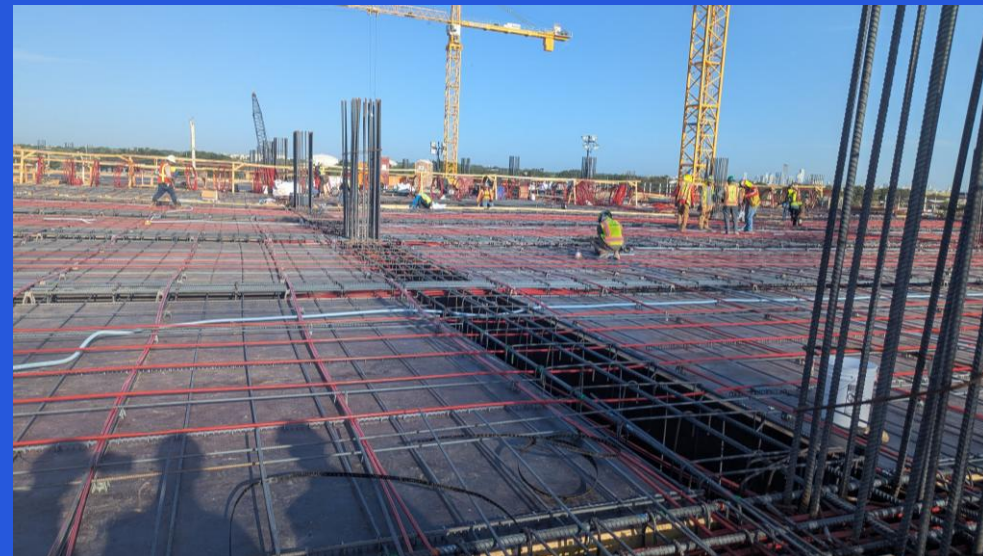
Garage deck with post-tensioned cables
