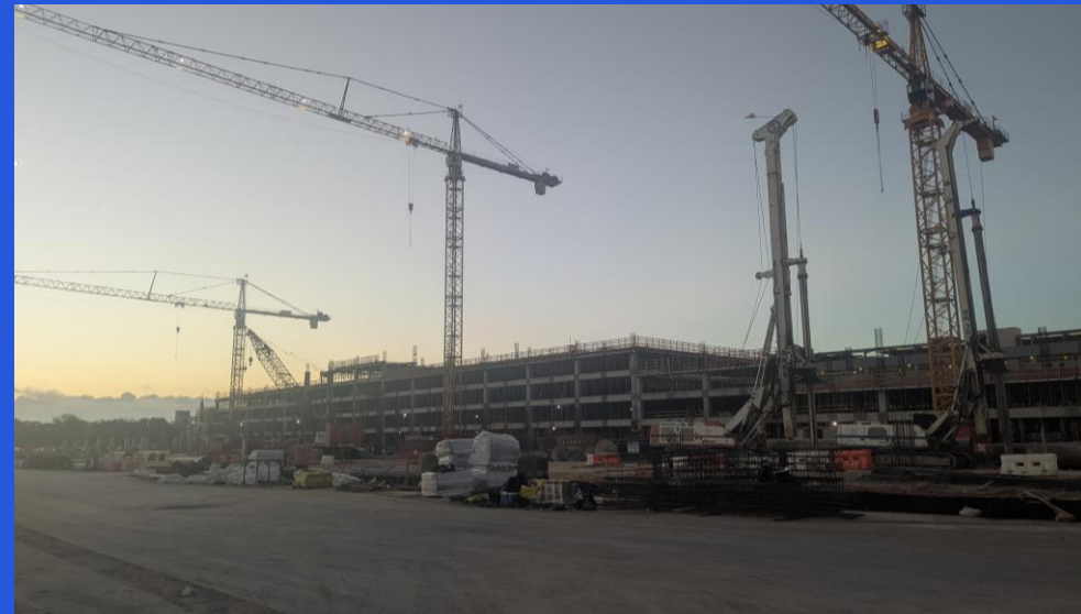
Garage viewed from the northwest including tower cranes
