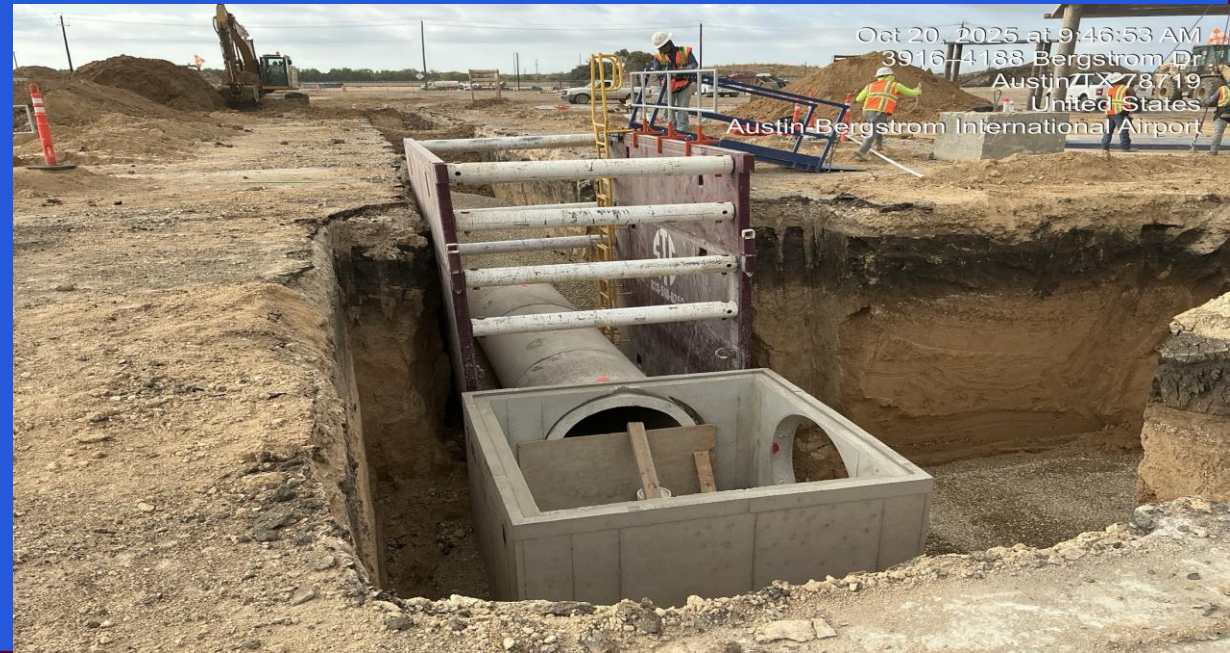
Phase 3 48" reinforced concrete pipe installation
