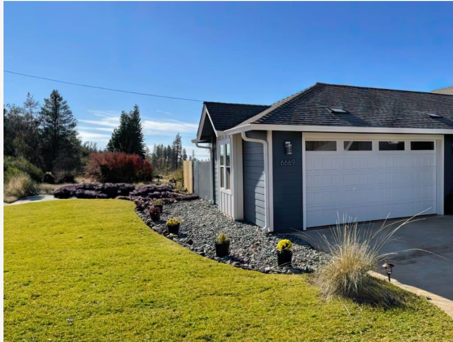
Placing landscaping away from buildings limits vegetation reflections and aligns with WUI code
