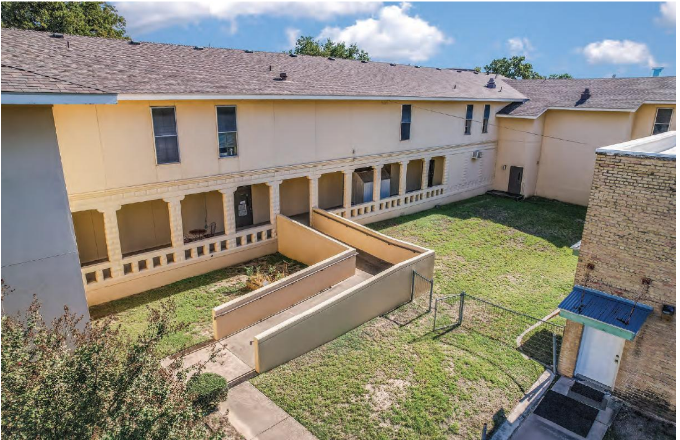
Interior courtyard of landmarked section of property, permit application, 2025
