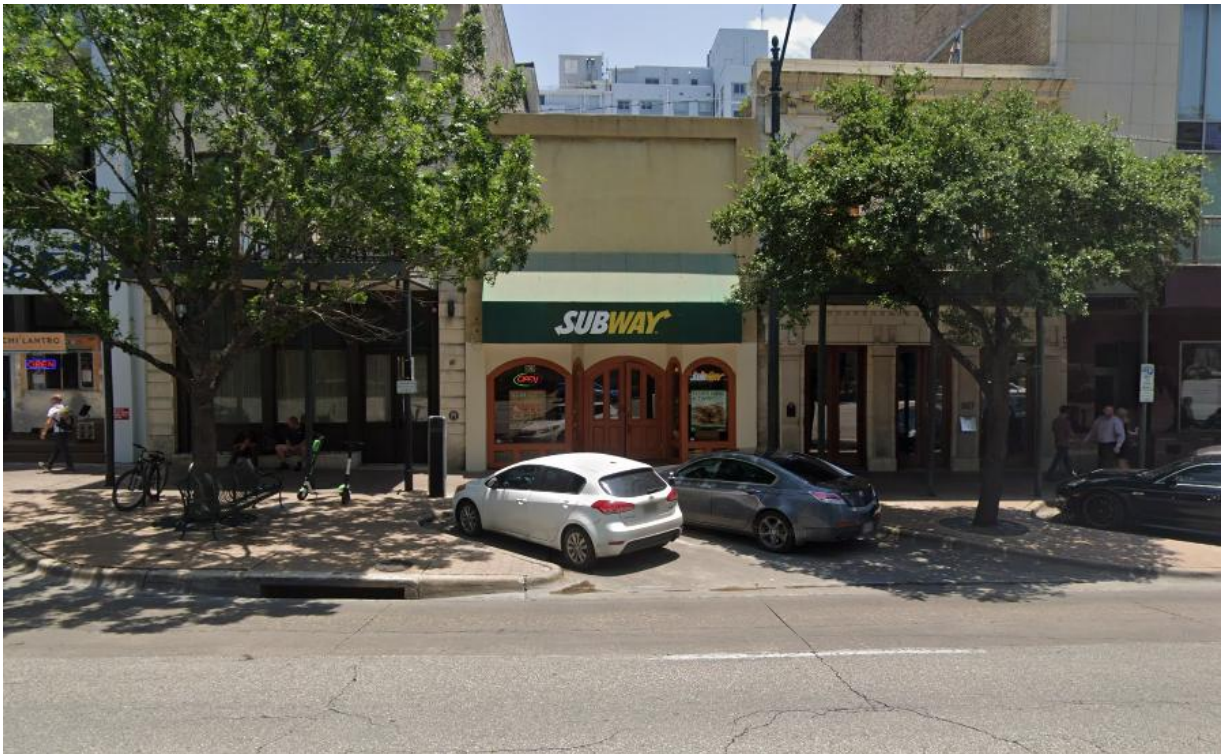
Google Streetview, 2019 (prior to removal of exterior stucco)
