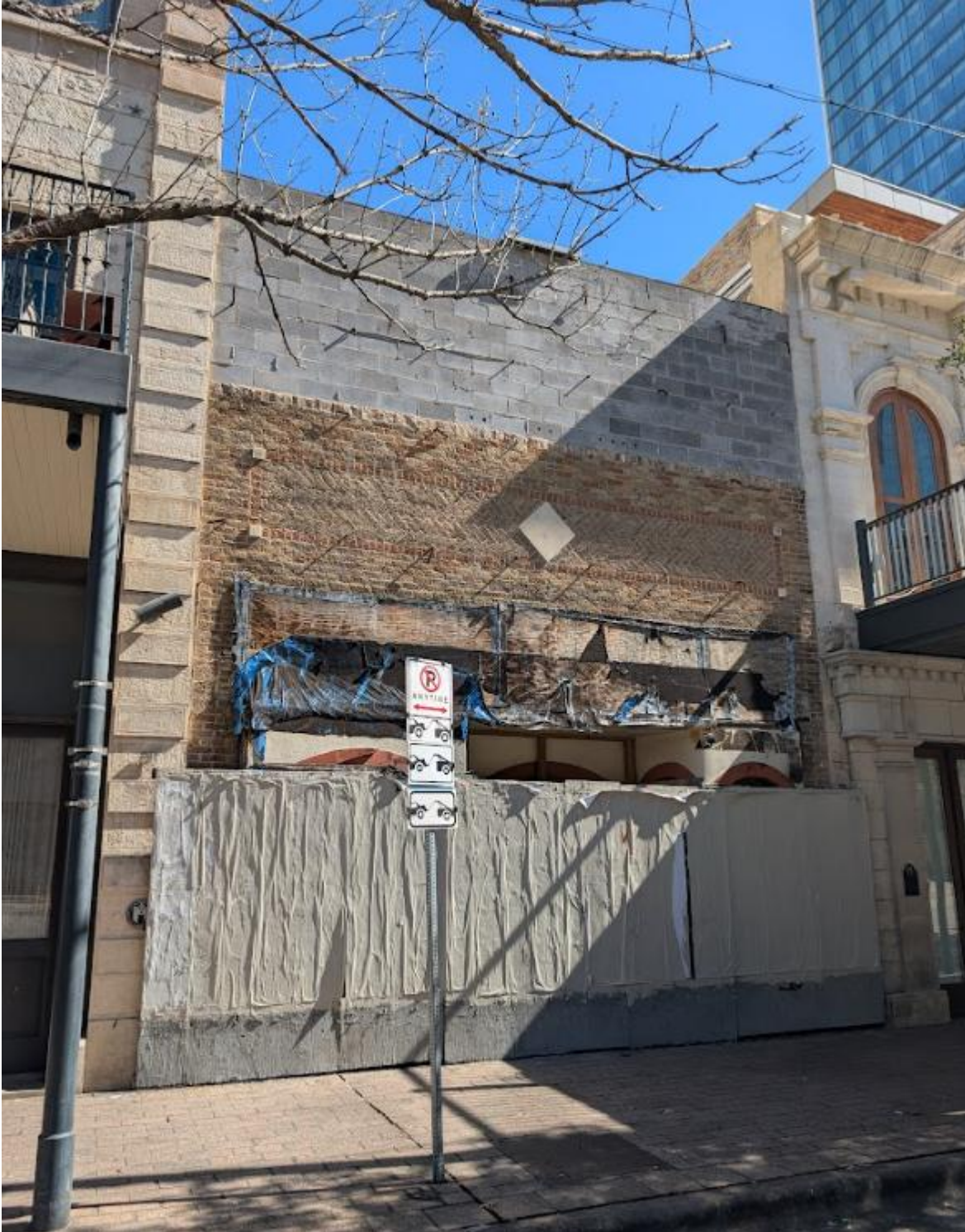
Site visit, February 2026
