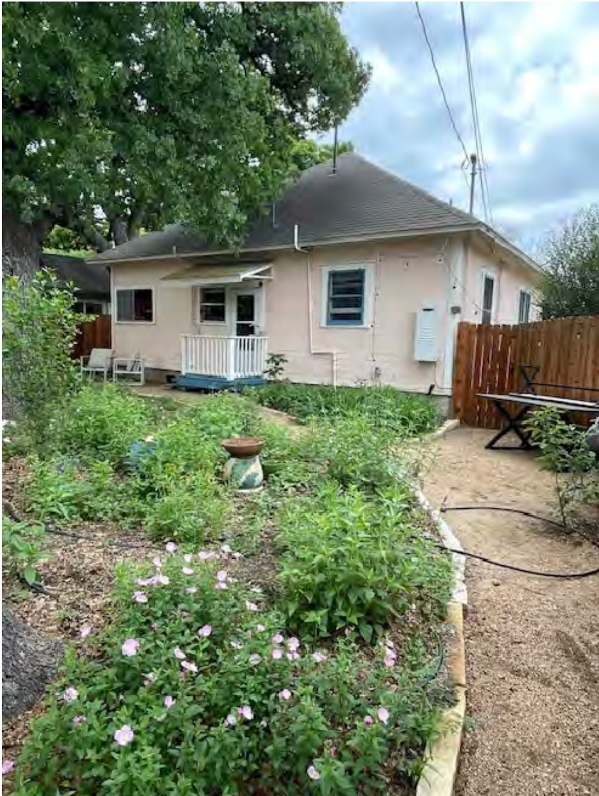
Photo 5: Caldwell House – North Façade
