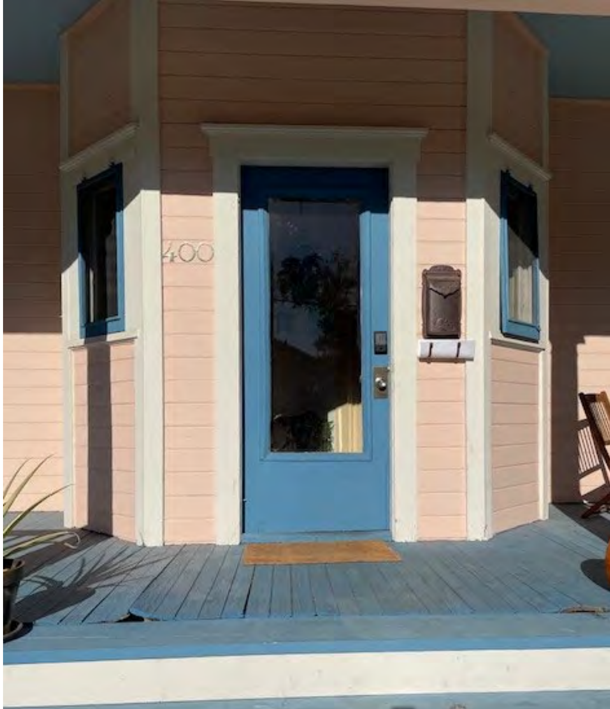
Photo 6: Caldwell House – Vestibule on Primary (South) Façade
