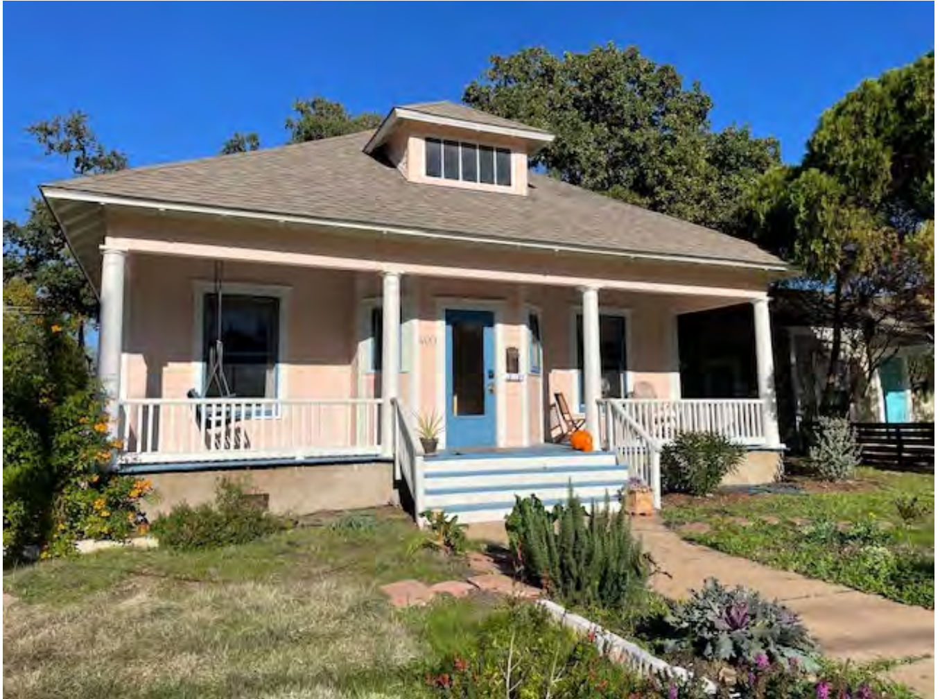
Photo 1: Caldwell House – Primary (South) facade
