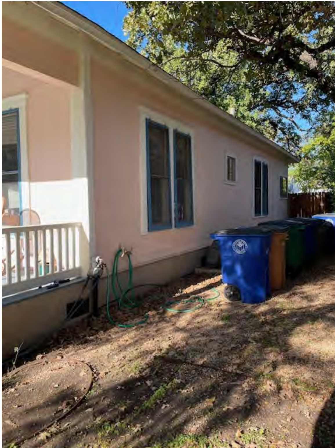
Photo 4: Caldwell House – East Façade
