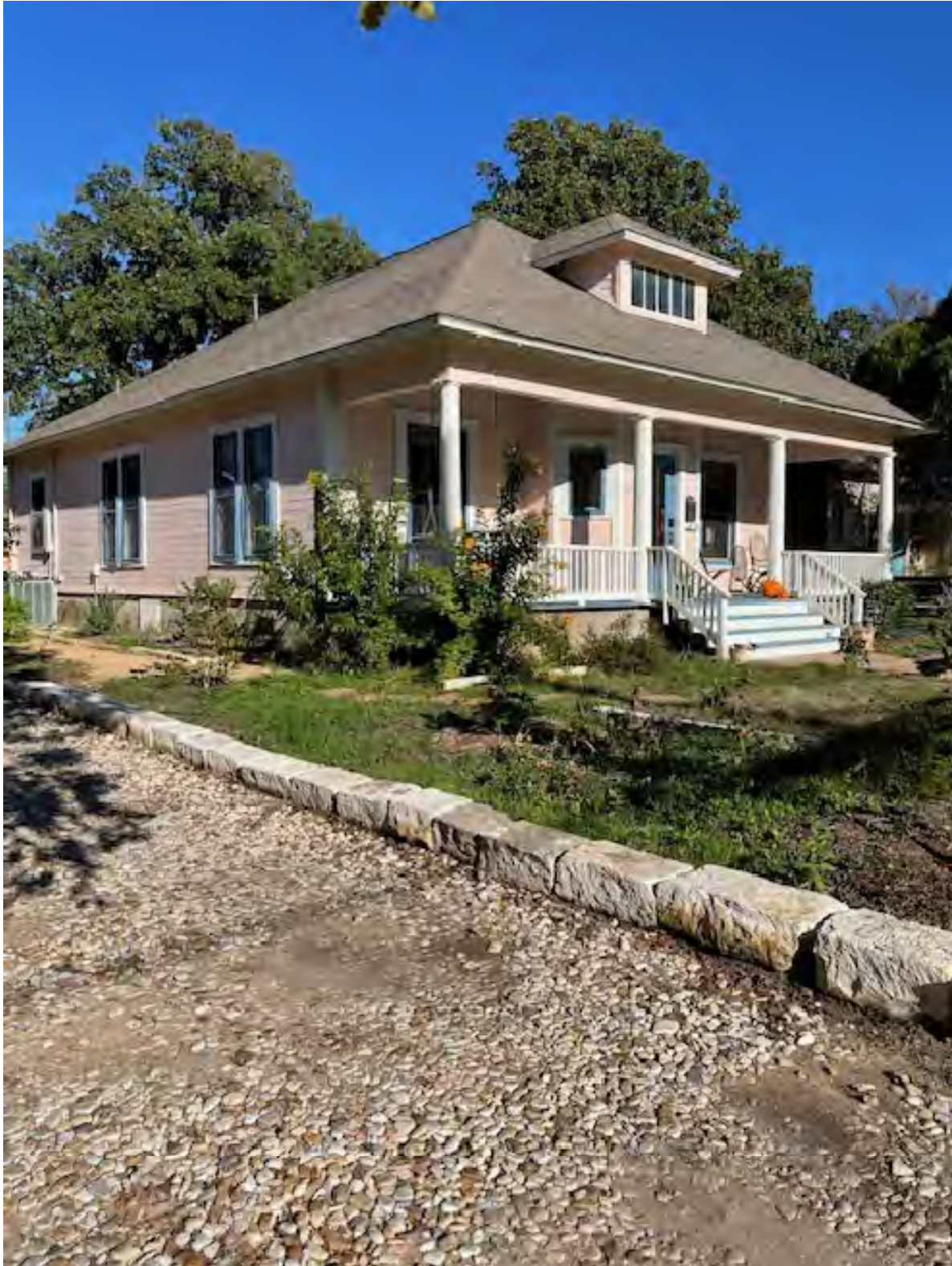
Photo 3: Caldwell House – West and South Facades
