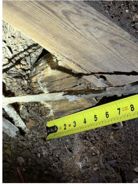
Figure 6. Timber pile foundation supporting the 4x6 timber beam – no concrete support was found.
