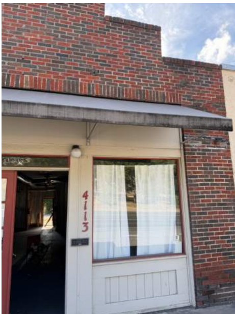
Figure 13. Existing front facade – storefront and brick parapet. The historic facade is to remain.
