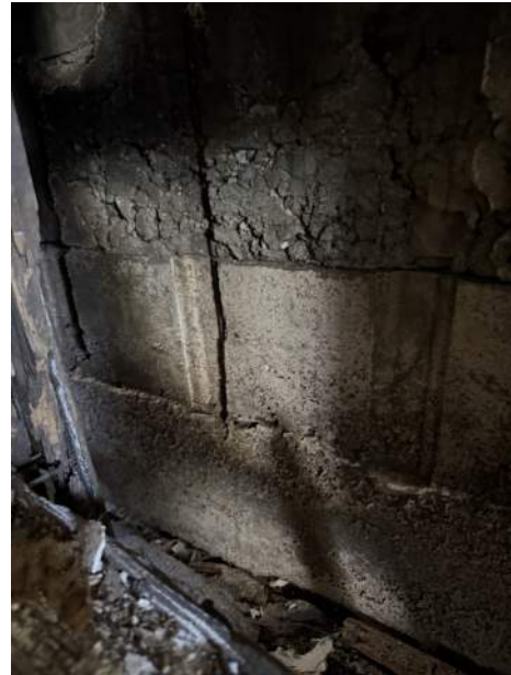
Figure 4. Exterior wall of the adjacent building to the south, viewed from the gap between the buildings.
