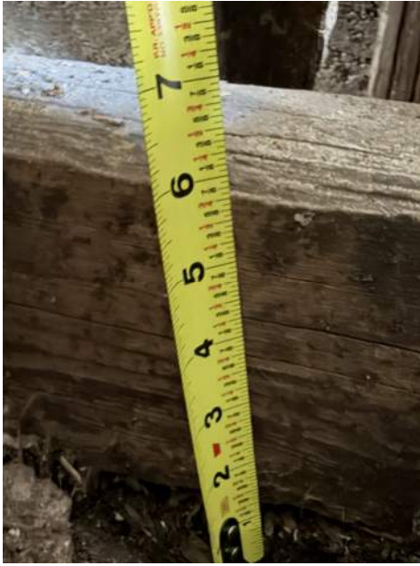
Figure 5. Existing 4x6 pressure-treated timber beam supporting the floor joists.
