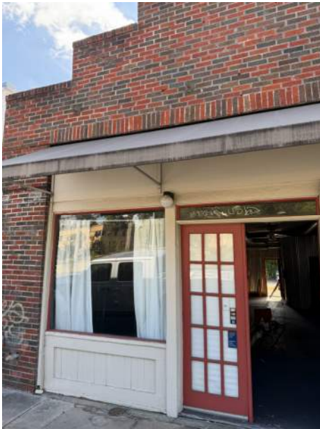
Figure 1. Existing front facade at Guadalupe Street – brick facade with storefront; the facade appears to bear on a concrete foundation.
