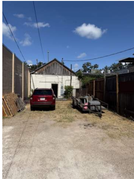
Figure 2. Rear of the existing structure – wood-framed building with paneled siding, set between adjacent buildings on each side.
