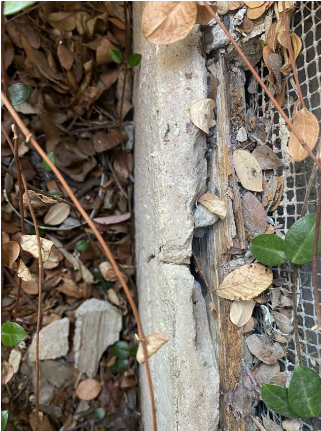
Photo 10. Detailed photo of a crawlspace vent along the eastern side façade of the main house, showing original wood siding underneath the stucco veneer. Photo dated March 12, 2026, by Emily Payne, HHM & Associates.
