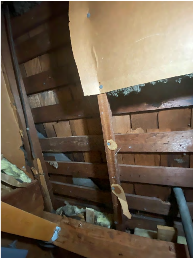
Photo 11. Detailed photo of the original wood roof shingles underneath the existing concrete tiles, taken from the interior of the attic, camera facing southeast, March 12, 2026. Photo by Emily Payne, HHM & Associates.
