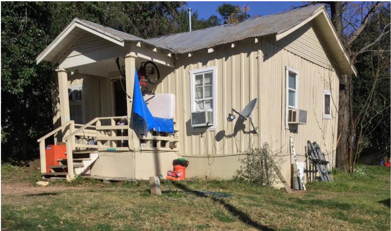
East Austin Historic Resource Survey, 2016. Note wood frame windows present at time of survey.
