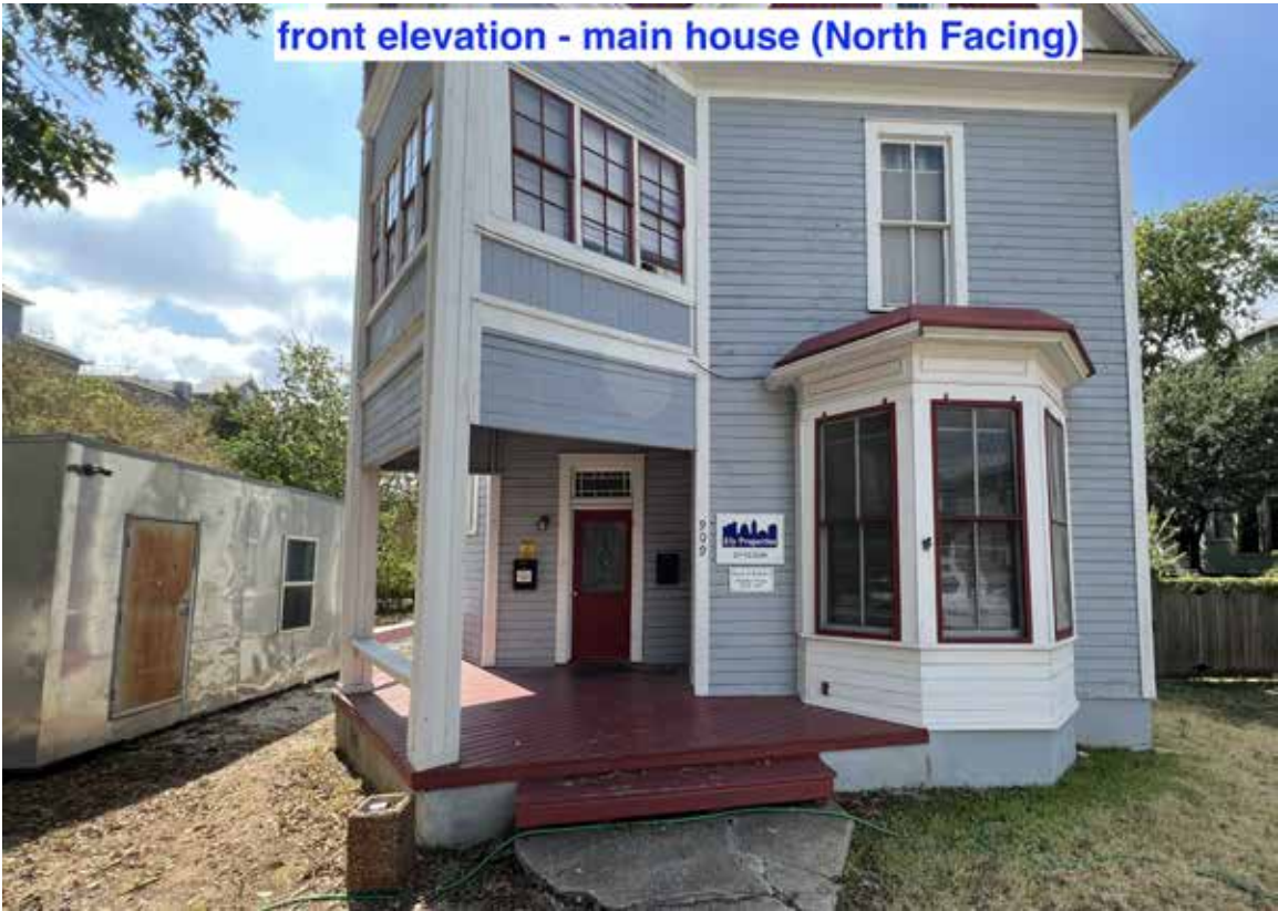
street elevation - main house (North Facing)
