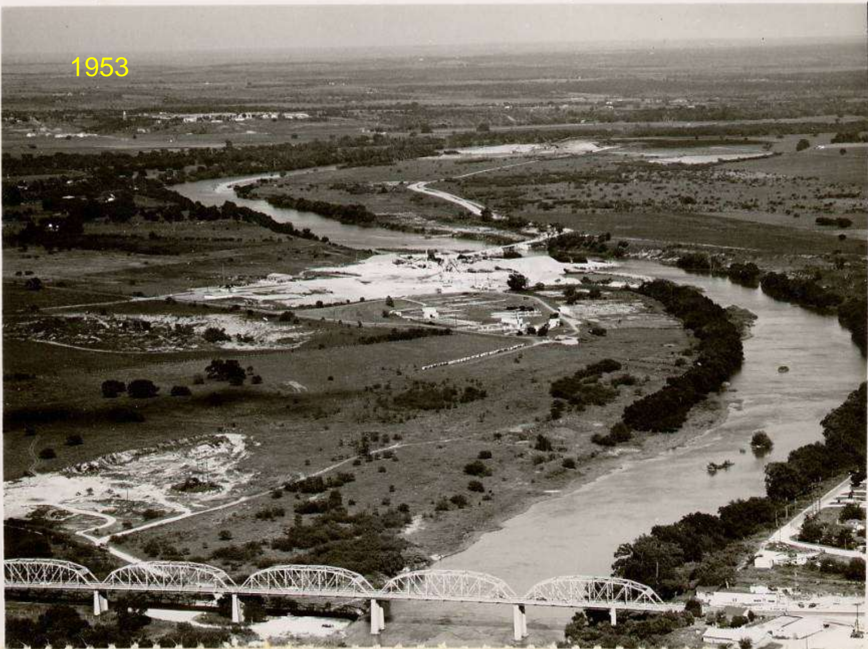
3402 Montopolis Bridge, Colorado River, south of Austin
